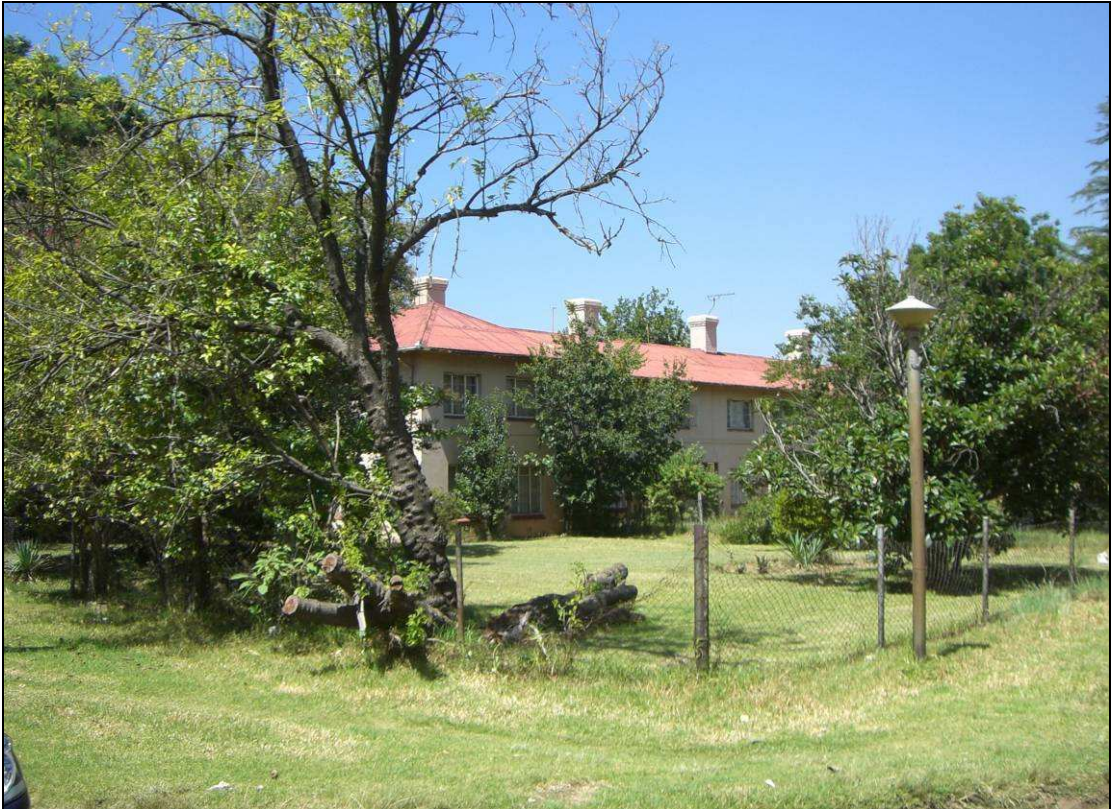
Plate 46 This image was taken before or during 2007 and appears to show the new married quarters building known in this report as Building 8. The photograph was taken from the north-east.
