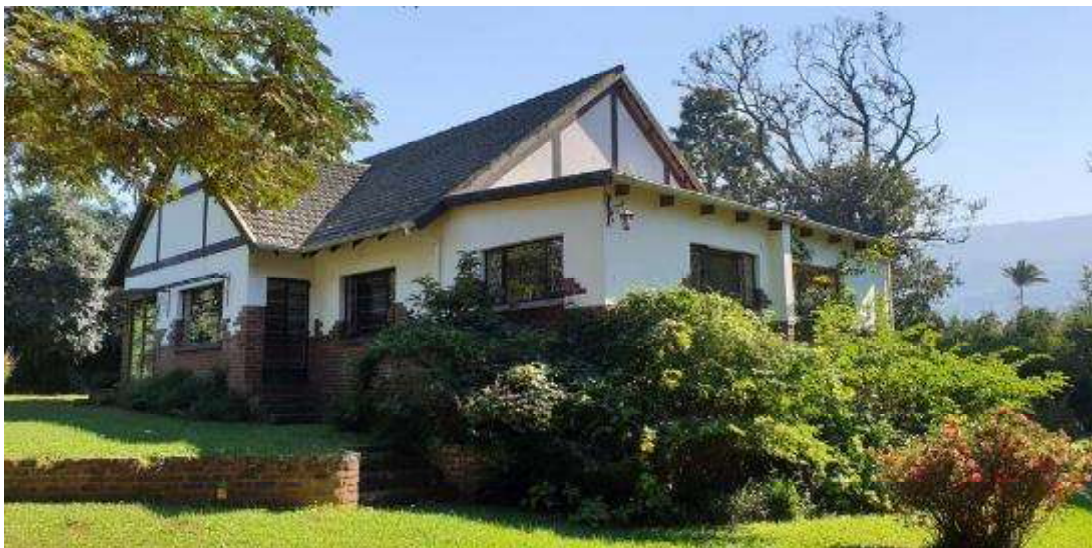
Photo 17. The Tudor Revival Style house at 635 Town Bush Road. The Victorian and Edwardian Tudor Style elements are apparent in the steeply-pitched roof; the wooden Tudor (stucco) decoration (half-timbering effect) on its upper walls; the half brick on its lower walls; and an overall suggestion of quaintness. Southern corner. Photo: courtesy Mr Ridwaan Essa.
