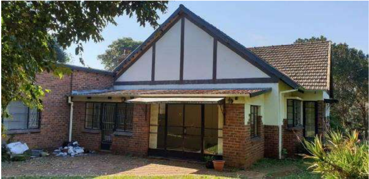
Photo 20: The western corner of the house. Note the stucco decoration is further reflected in the glass doorways, and windows so typical of this style. Also note the tall, rather narrow windows, in a simulation of the Gothic Style, typical of the Tudor Style; and of the jutting, and stepped side façade of the house, in the creation of an impression of bay windows, as well as the actual bay window. Western corner. Photo: courtesy Mr Ridwaan Essa.
