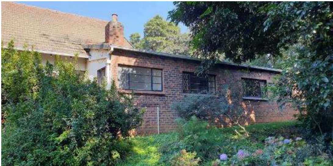
Photo 19. The eastern façade of the Tudor Revival home. Note the high rather ornate brickwork chimney with a chimney pot. This is very typical of the Tudor Revival Style, and of Edwardian homes as a whole. The reddish brickwork is also very typical of historic homes in this region, even though it is not of the old salmon-coloured brickwork seen during the deep Victorian and Edwardian period in this area. Photo: courtesy Mr Ridwaan Essa.
