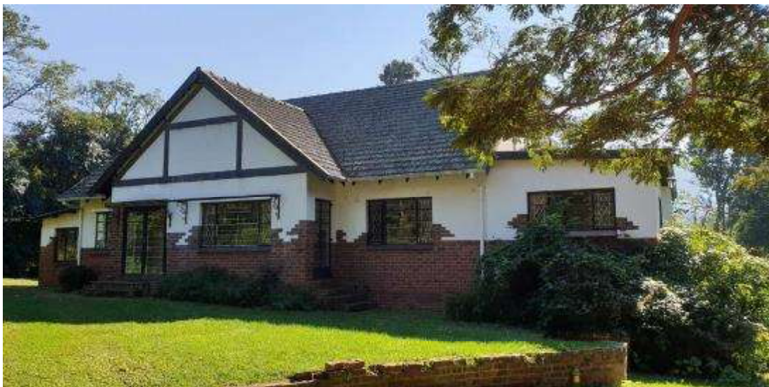
Plate 16. Another photograph of the Tudor Revival Style house snugly wrapped in shrubbery to the one side. Photo: Courtesy Mr Ridwaan Essa.
