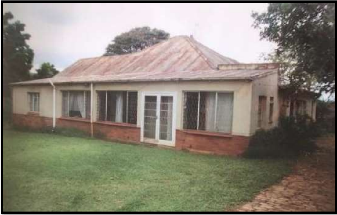
Plate 10. A better view of the same side of the house, but without the chimney. The rambly, ad-hoc, and organic style of the house is typical of influence from the Picturesque Movement in house styles, discussed earlier in the text. A building does not have to be symmetrical, or beautiful, to be considered heritage. Photo: courtesy Mohammed Moosa.
