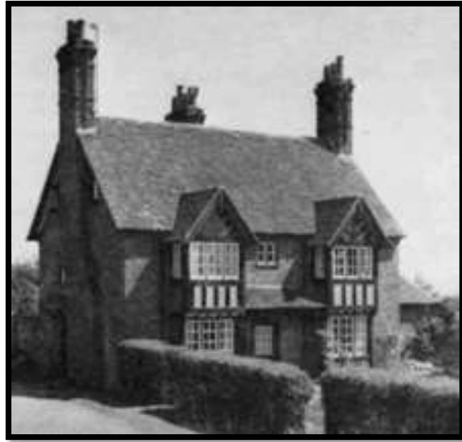
Photo 23: Built circa 1870 two semi-detached cottages at Mentmore appear as one Tudor style house. Source: Wikipedia.
