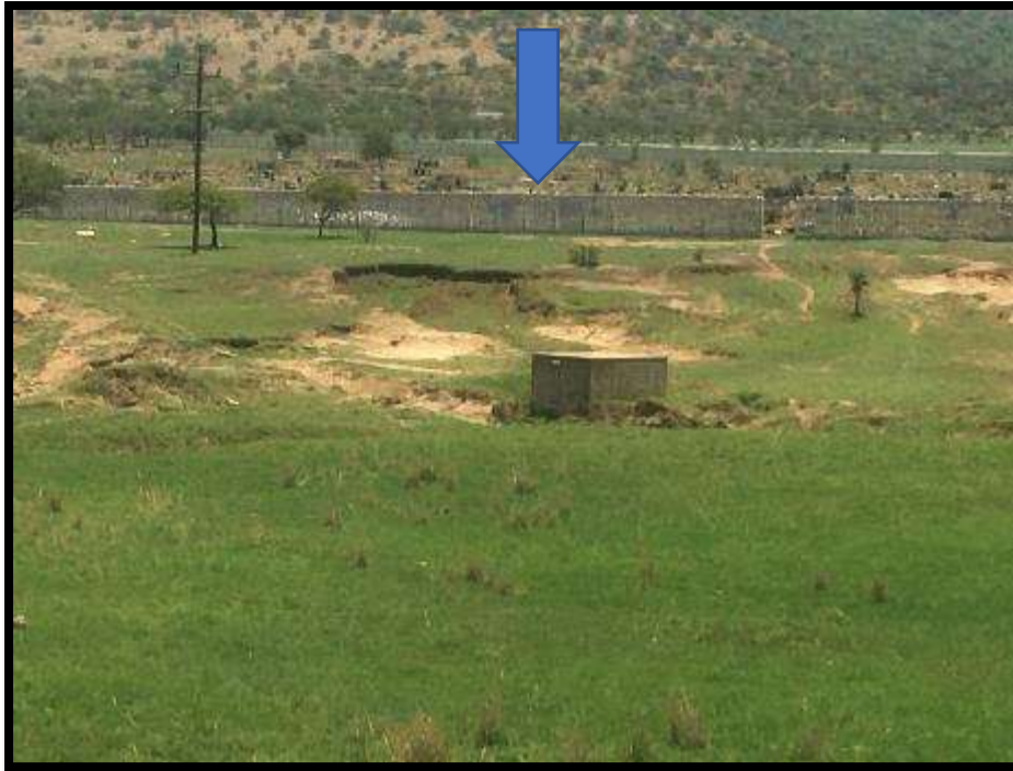
Figure 11. A large cemetery is situated directly adjacent to the proposed pipeline trajectory (north bank). However, it is well demarcated and protected by a concrete fence.
