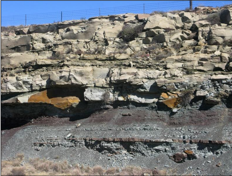
Fig. 8. Package of pale brown, tabular-bedded channel sandstones of the Katberg Formation with markedly gullied base incising colour-banded overbank mudrocks, road cutting along the N10, Farm RE1/1 (Loc. 127).
