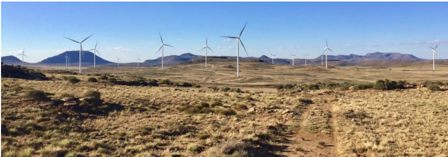
Figure 6. The nearby established Noupoort wind farm reflects how the Phezukomoya landscape will change.
