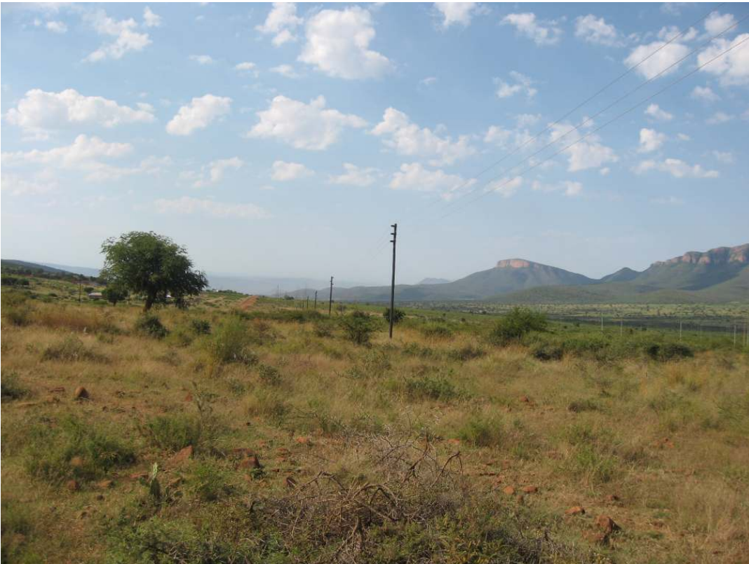
Photo 4: View of the power line from the north.
