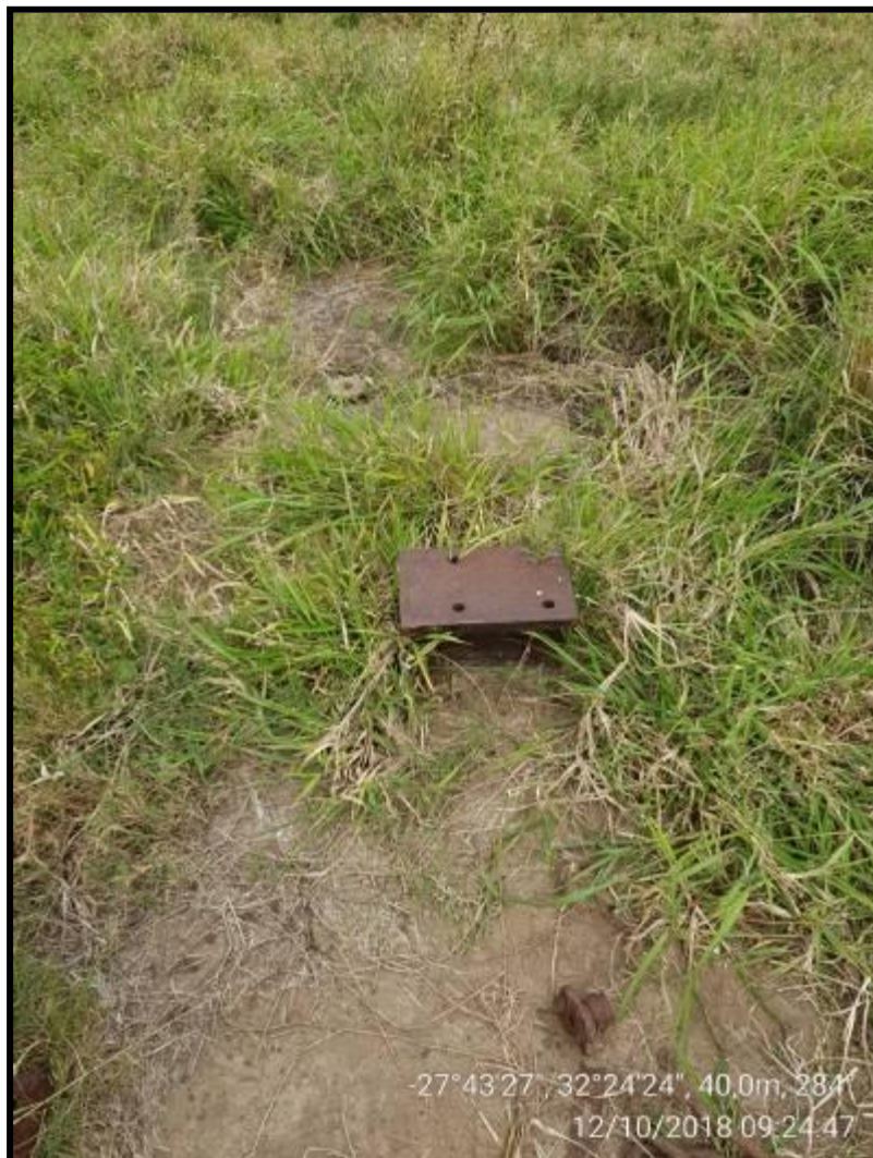
FIG. 94: FOUNDATIONS AT PND052
