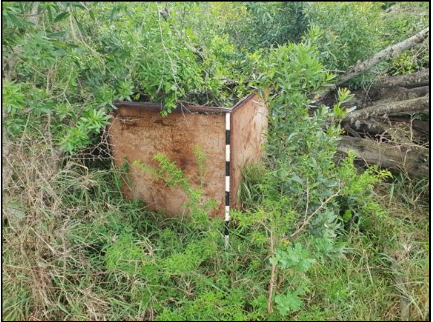
FIG. 82: STORAGE TANK AT PND050
