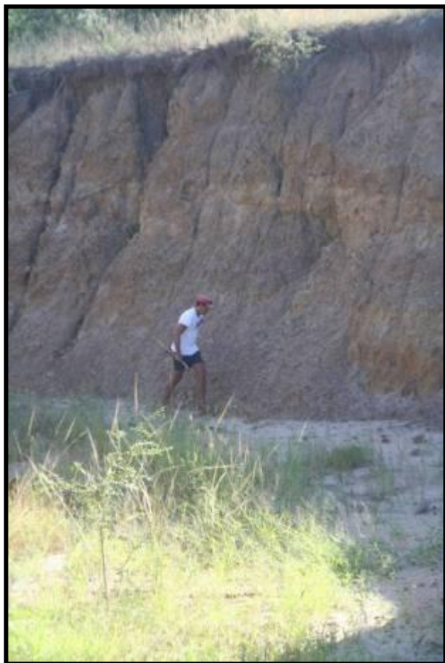
FIG. 53 EMBANKMENT AT PND035
