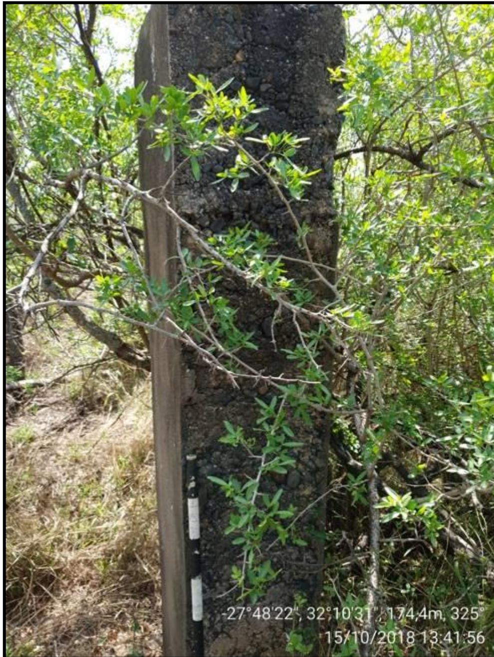
FIG. 112: FOUNDATIONS AT PND064
