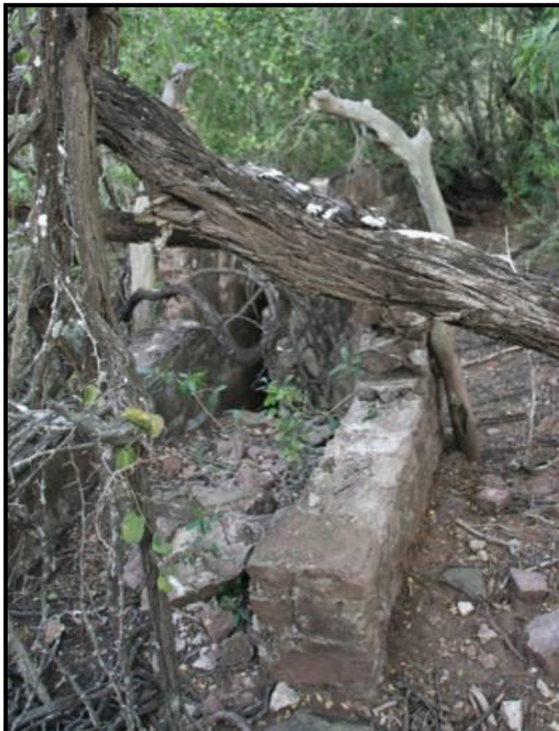
FIG. 60: WATER TROUGH AT PND039
