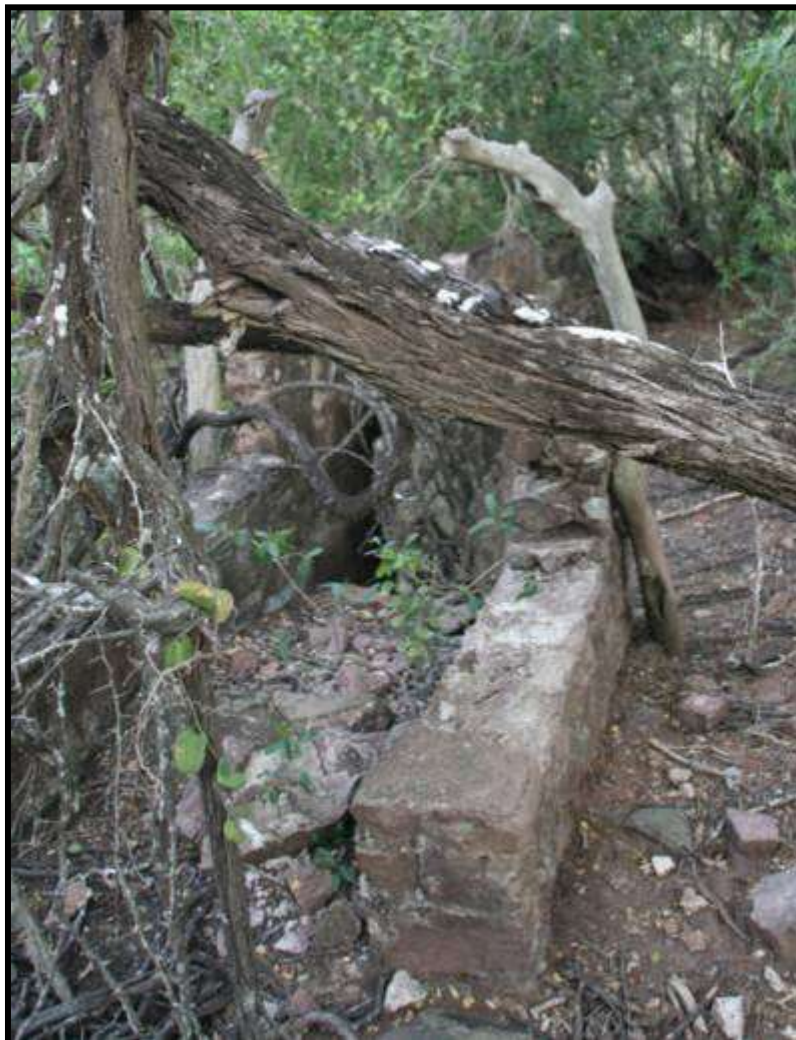
FIG. 60: WATER TROUGH AT PND039
