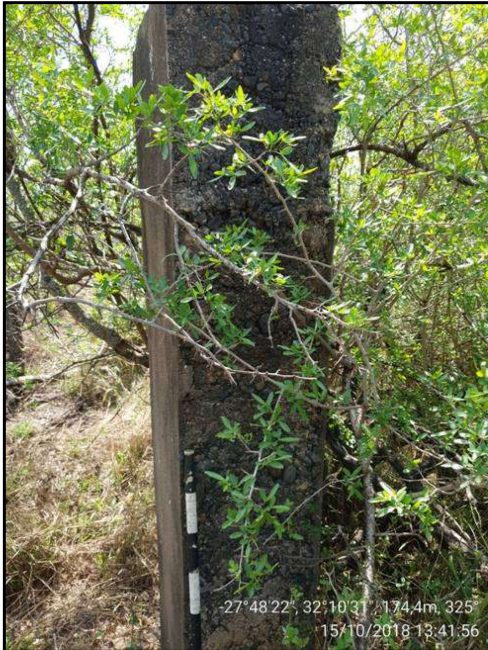
FIG. 112: FOUNDATIONS AT PND064
