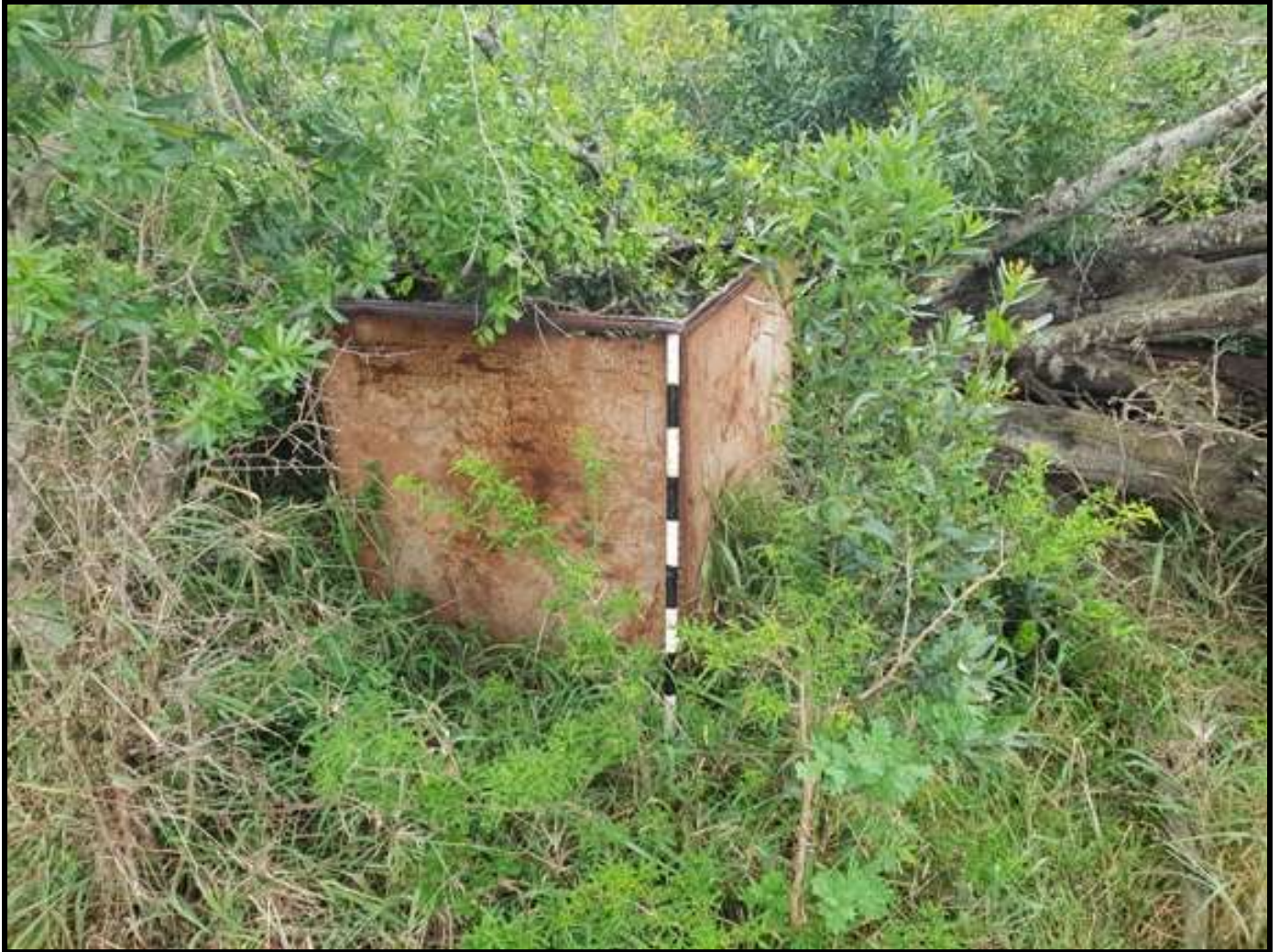
FIG. 82: STORAGE TANK AT PND050
