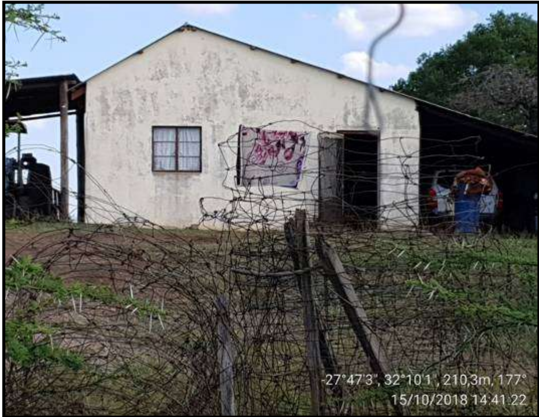
FIG. 143: BUILDINGS AT INGAGALU (PND084)
