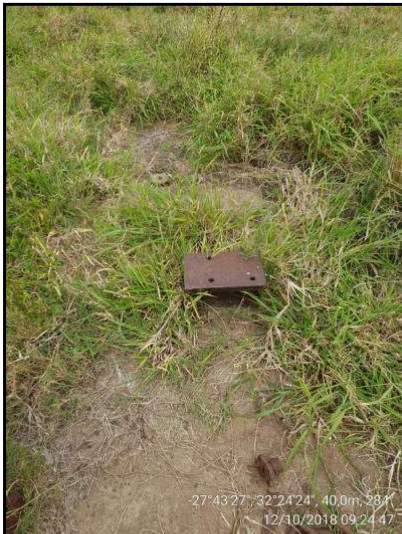
FIG. 94: FOUNDATIONS AT PND052
