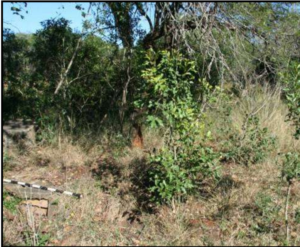
FIG. 56: HOUSE FOUNDATIONS WITH PILLAR AT PND037
