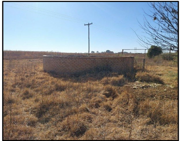
Figure 7.20. Structure at PF0002.
