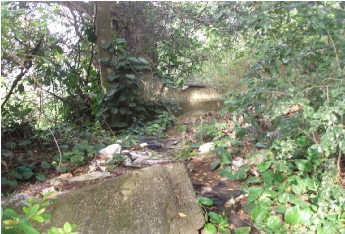
Figure 13: Remains of concrete structure
