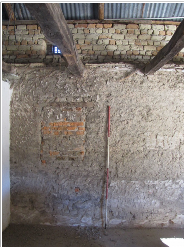
Plate 3: Eastern elevation. Stone-built wall 01 up to 200mm; overlain by wall 02 with window; window blocking 17; overlain by roof support 19. View to south-east, 2.0m scale.
