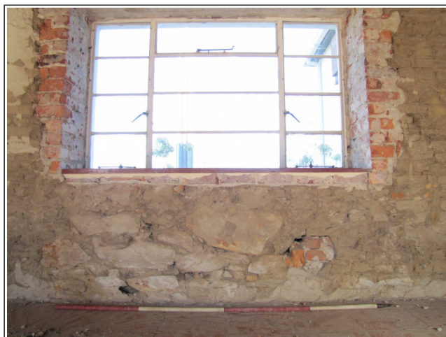
Plate 2: Stone-built wall 01 along eastern elevation. Shows wall 01 (centre) was originally built to higher level along the side building walls than the 150mm high footing continuing to either side; overlain by sun-dried brick wall 02; both truncated by red-brick window 06. View to south-east.
