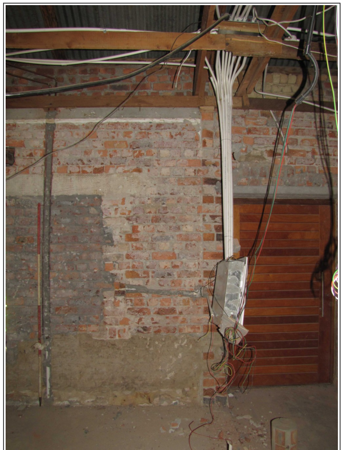
Plate 5: Western elevation showing structures from Phases 5 and 6. Note the more lime-based cement used in Phase 5 (centre) compared to the grey cement of Phase 6 window blocking on left. View to north-west, 2.0m scale.
