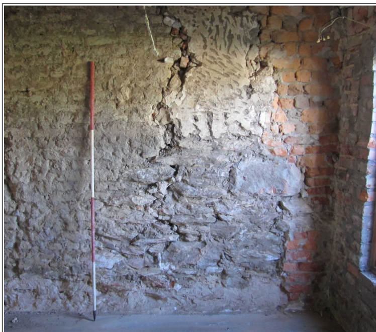
Plate 1: North-west corner of building: sun-dried brick wall 02 on the left; overlying the robbed edge of stone-built wall 01 in the centre; which is overlaid by red-brick gable wall 03 on the right. View to the north-west.
