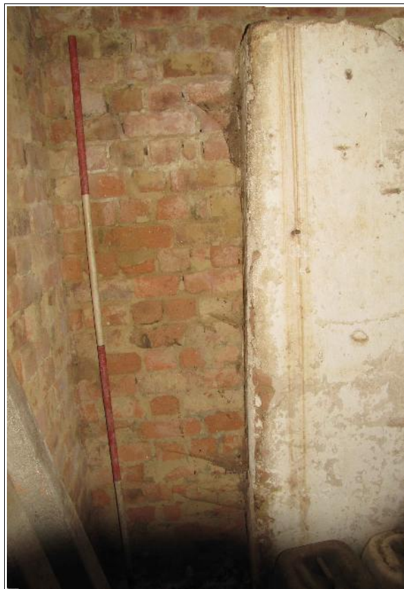
Plate 2: Section 10 showing interface between walls 25 and 26.
