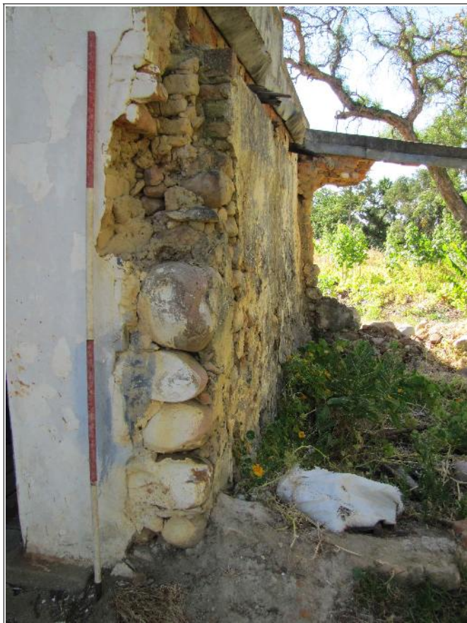
Plate 1: Photograph showing keyed-in continuation of wall 26 to the north.
