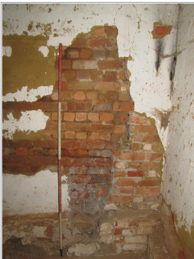
Plate 7: Section 11 showing end gable wall 31 overlying stone-built wall 27.
