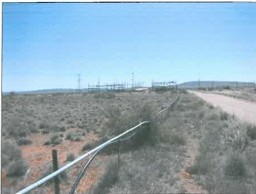
Fig.1 Garona substation on the Sishen-Saldanha railway line.
