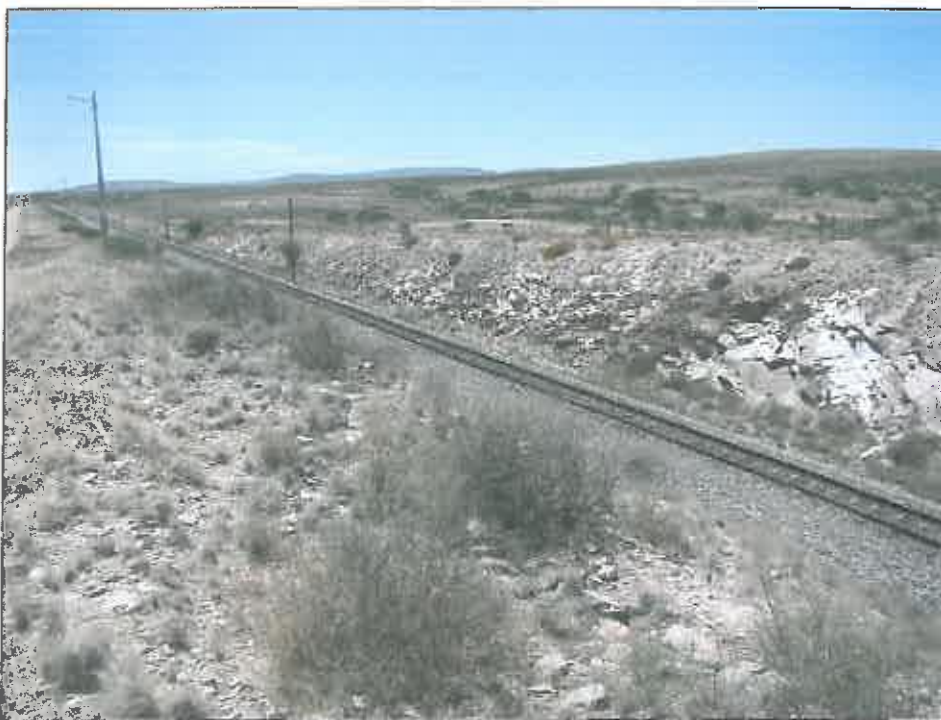
Fig.13 Point C along the railway line from Garona to Sanddraai.
