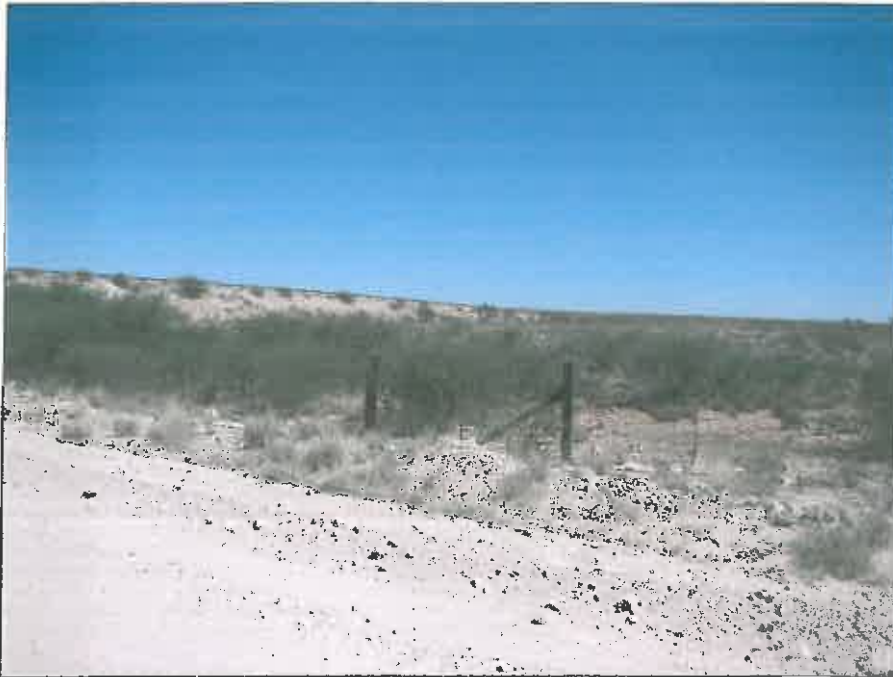
Fig.10 Point B along the railway line from Garona to Sanddraai.
