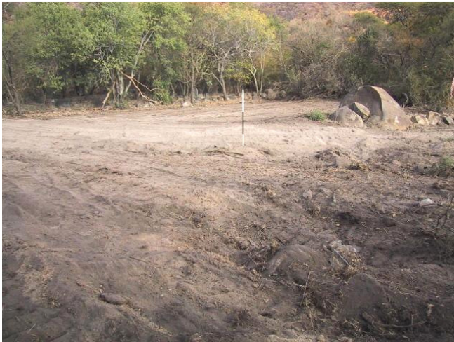
Fig 9. Leveled area, site 1
