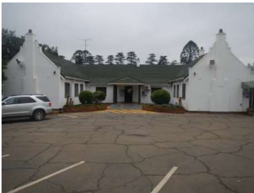
Figure 11: Front façade of the first old building currently being used as offices. Notice the steep roof near the gables on either side. The façade of the house is strongly reminiscent of Victorian period houses
