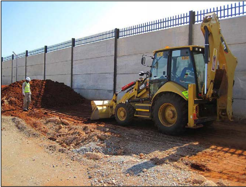
Figure 11: PGS staff supervising the TLB during the removal of the over burden and top soil.
