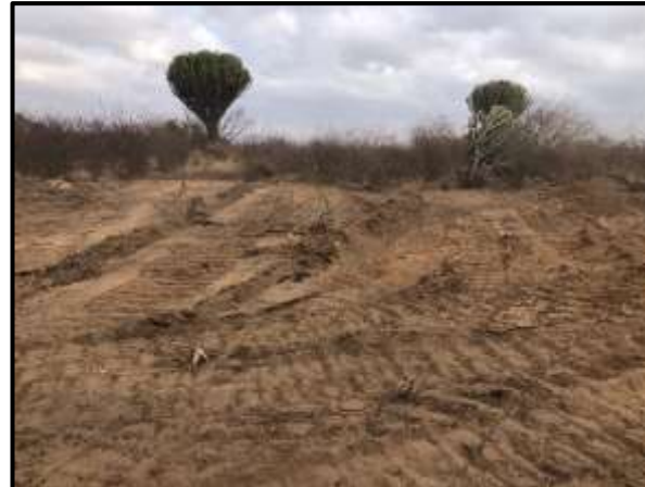
Figure 6-5: Area after clearing.
