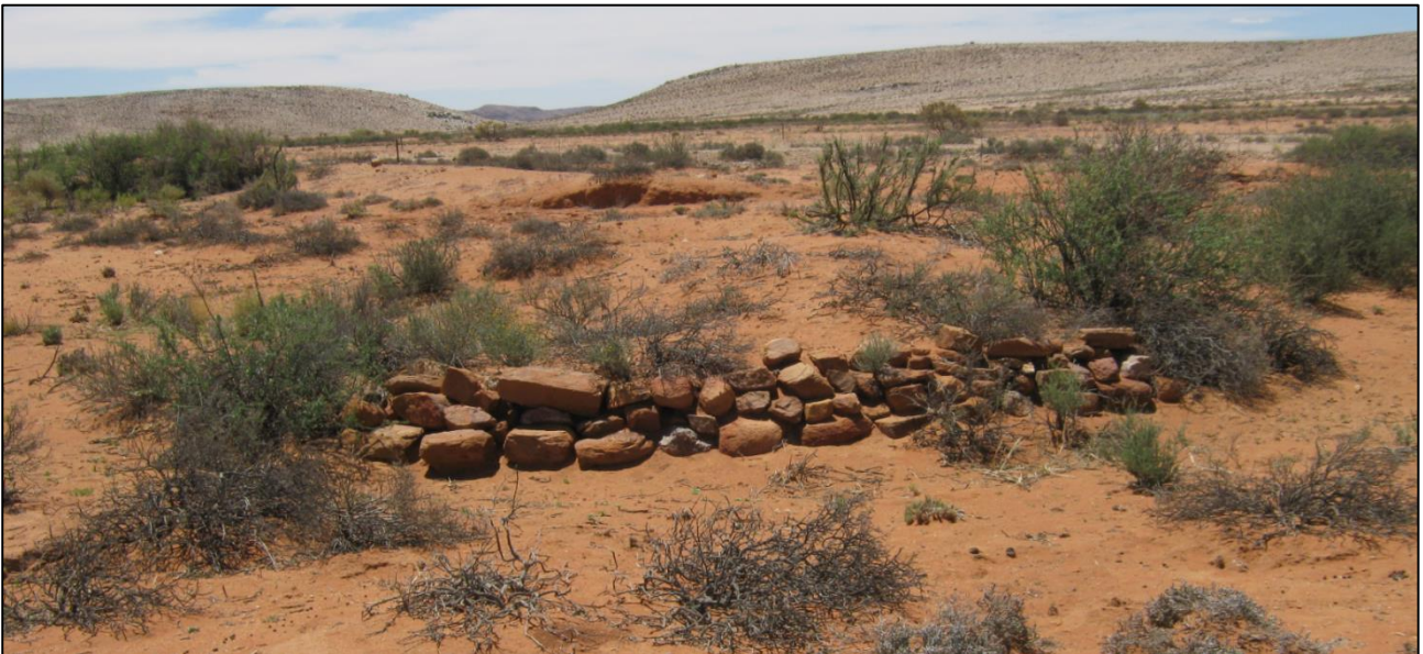
Figure 26: Earthen dam with end walls at waypoint 566.
