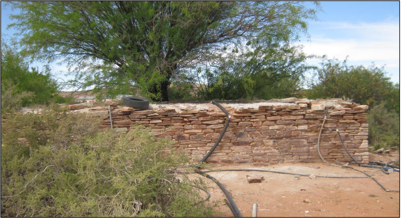
Figure 32: Stone-walled water reservoir at waypoint 526.
