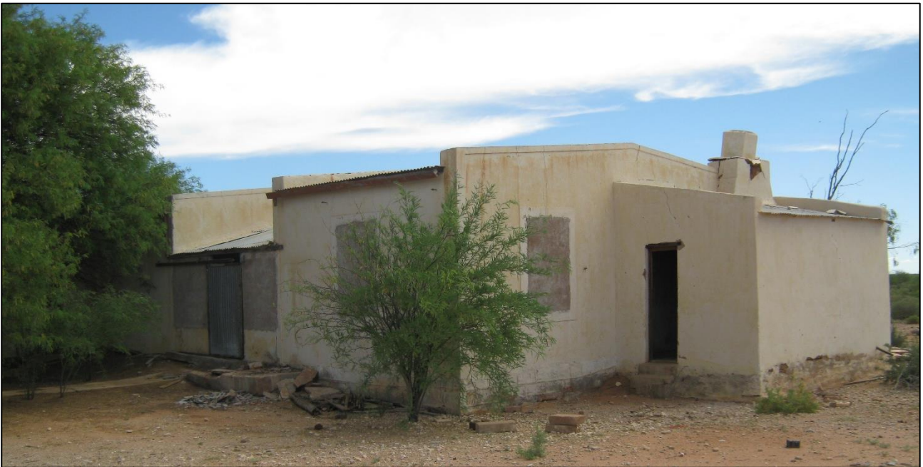
Figure 30: Structure with bricked up windows at the farmstead ay waypoint 526.
