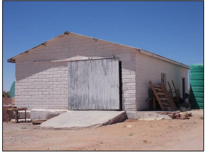
Figure 34: Outbuilding of decorative breeze blocks at LZM2012/002 (point 086). It is likely also 1940s in age.
