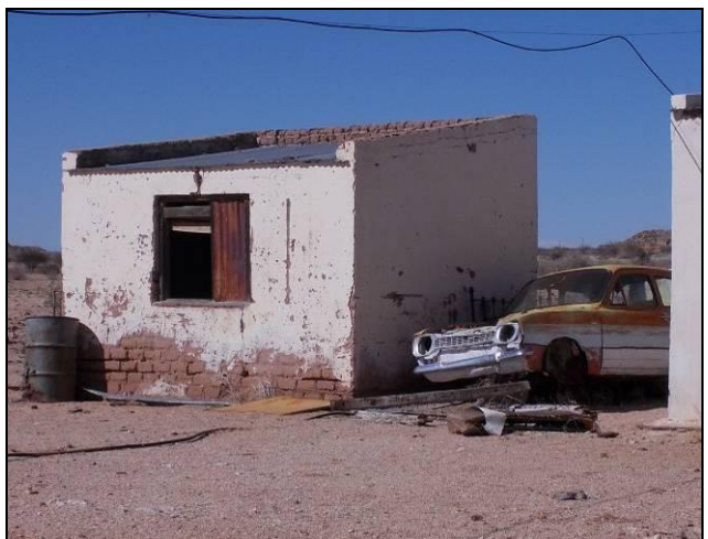
Figure 32: Close up of one of the YAS2012/004 houses showing its construction to be of locally made, sun-dried bricks.
