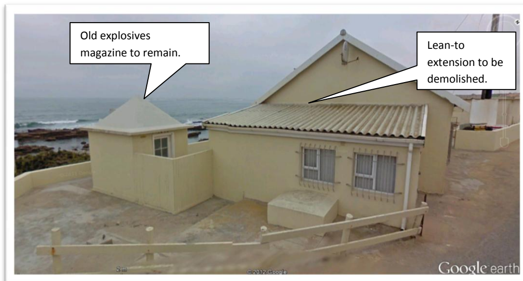
Figure 3 The structure which is the subject of this enquiry. The lean-to extension to the building requires demolition. View is from south to north. The pitched roof bungalow and magazine is to remain.
