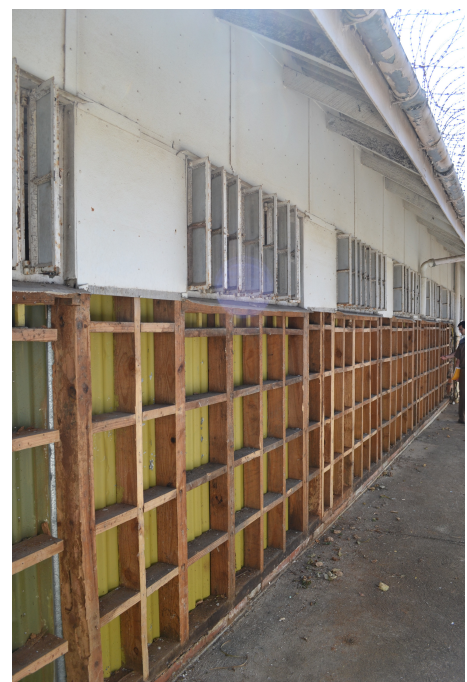
Photo 4. Timber-framed construction Blocks 6 & 7, partly exposed.
