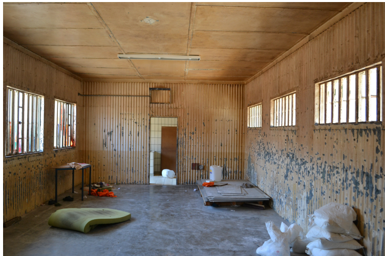
Photo 7. Interior of a Communal Cell Blocks 6 & 7.
