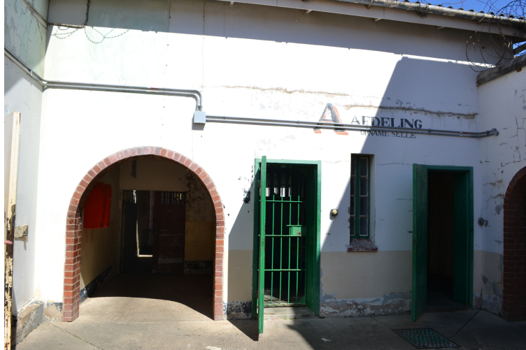
Photo 6. South side of Block 4
