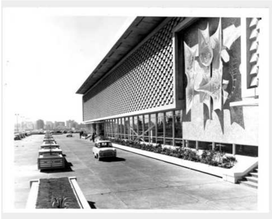
Figure 6: Exterior of the passenger Terminal , OTB: 1963
