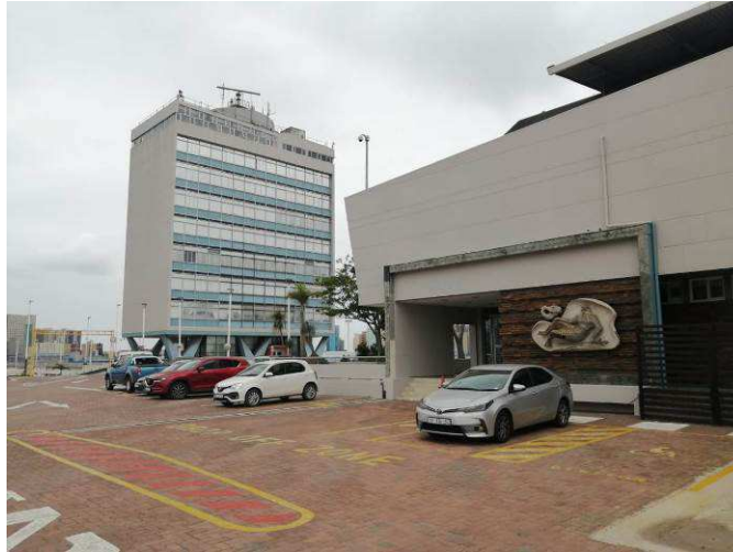
Figure 19: Exterior View of Ocean Terminal Entrance November 2020
