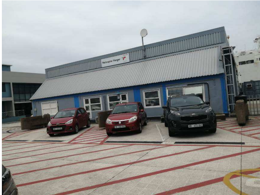
Figure 13: TNPA Helicopter Hangar adjacent OTB
