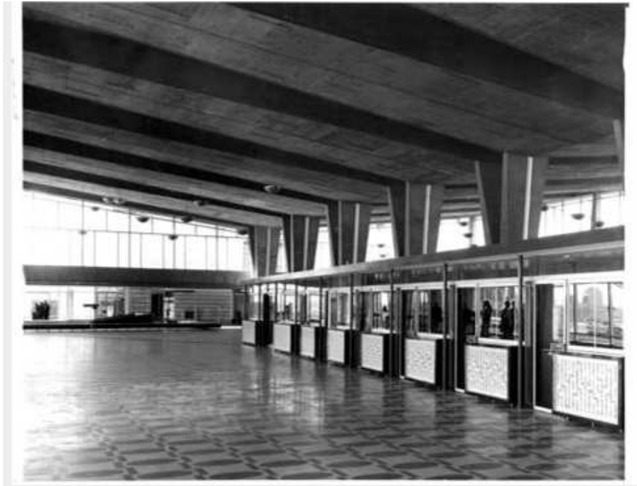
Figure 154: Double volume interior with Y columns and concrete roof
