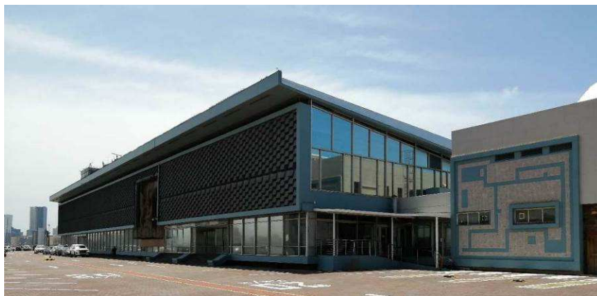
Figure 18: Exterior OTB : Nov. 2020
