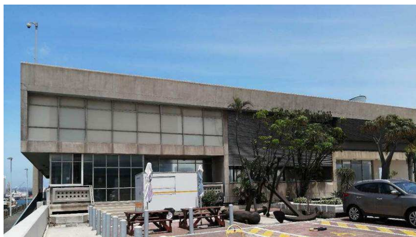
Figure 16: Exterior exposed concrete : Nov. 2020
