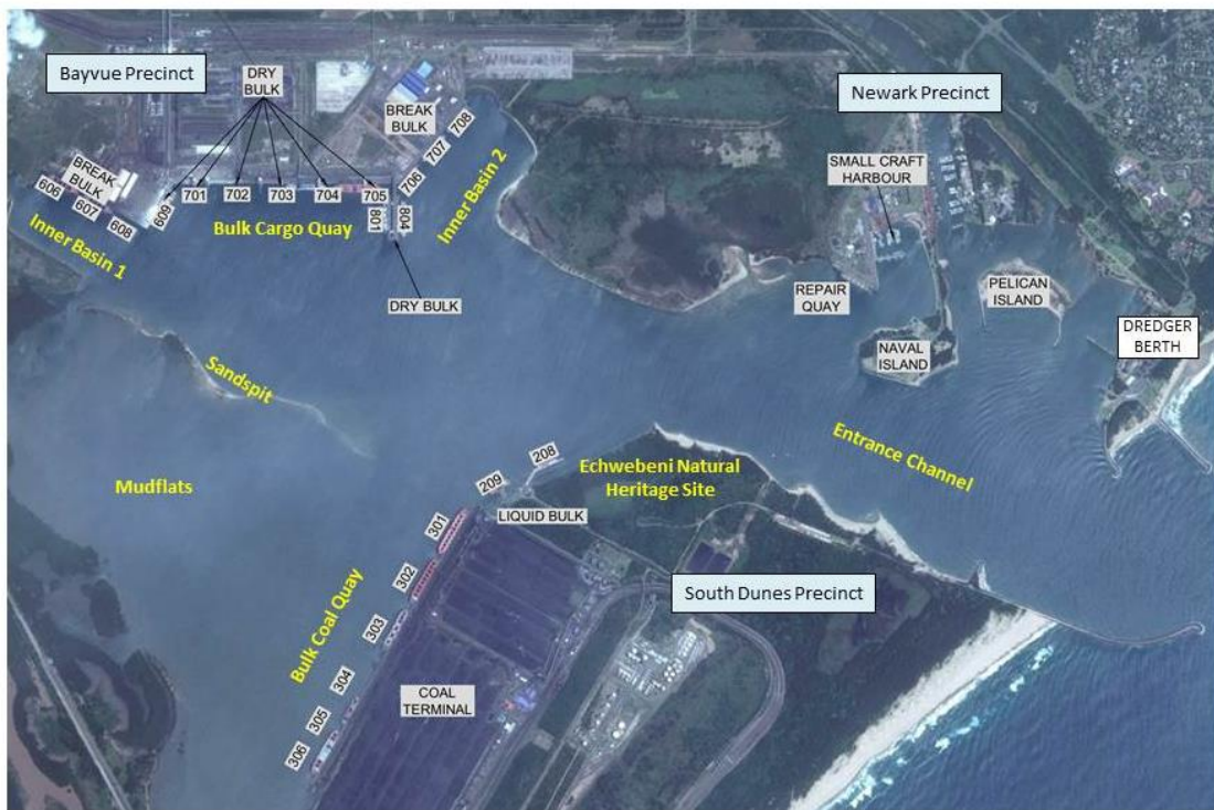
Figure 2.1: The existing layout of the Port of Richards Bay (Source: GoogleEarth, 2015).
