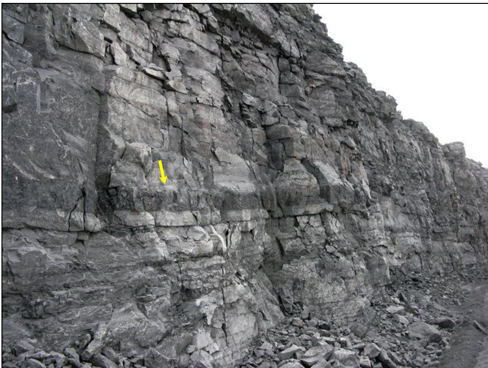
Fig. 32. View of cut face on the western side of the active northern pit at Lime Acres Quarry showing vertical section through the tabular-bedded Kogelbeen Formation limestones (Lime Acres Member) including the dark, c. 30 cm thick upper stromatolite marker bed (arrowed).
