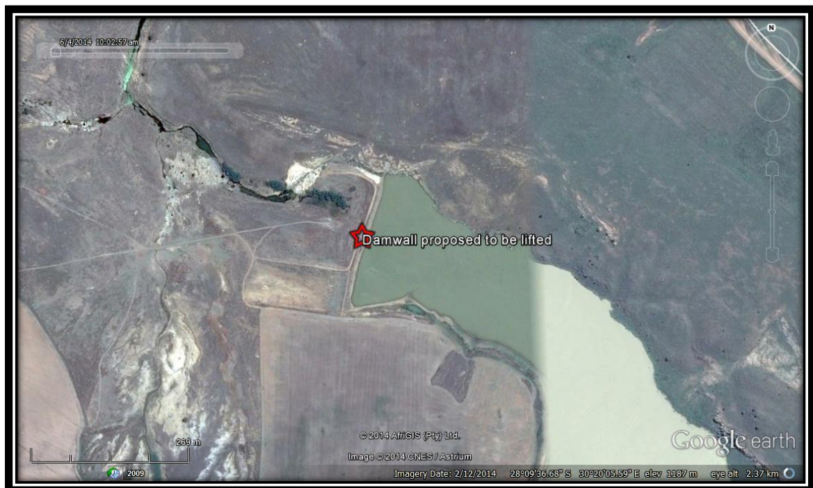
Figure 2. Google aerial photograph showing the location of the dam wall proposed to be lifted.
