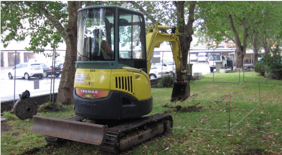
Figure 27 David Halkett (ACO) commences excavation on SI01
