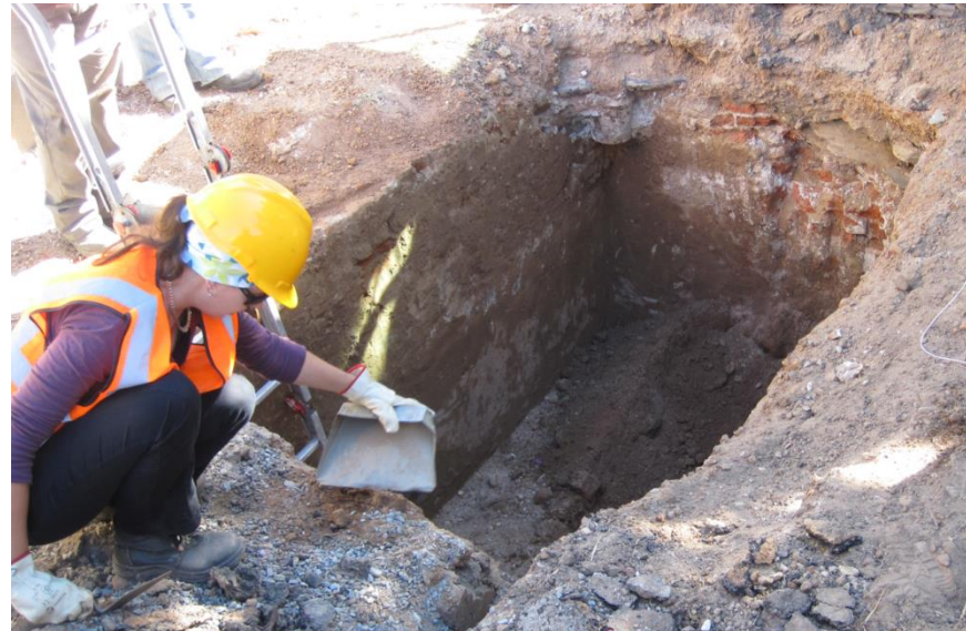
Figure 16 The brick work and lime cement mortar construction of the vault is clearly visible.
