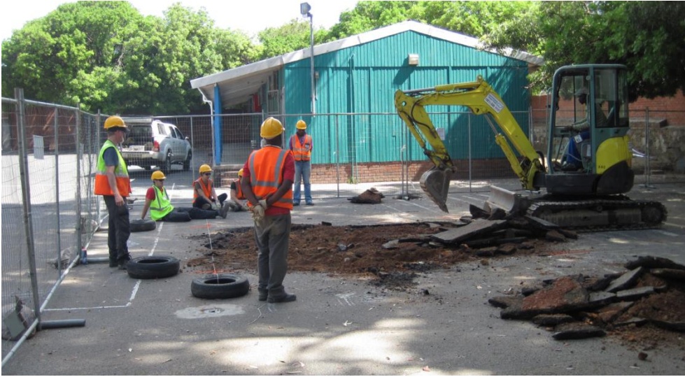
Figure 20 Commencement of Excavations at Prestwich School
