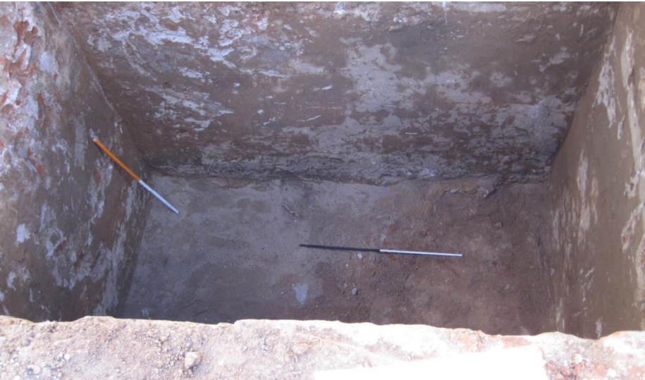
Figure 17 Vault at PTL 4 after it had been fully excavated to its shale slab floor.
