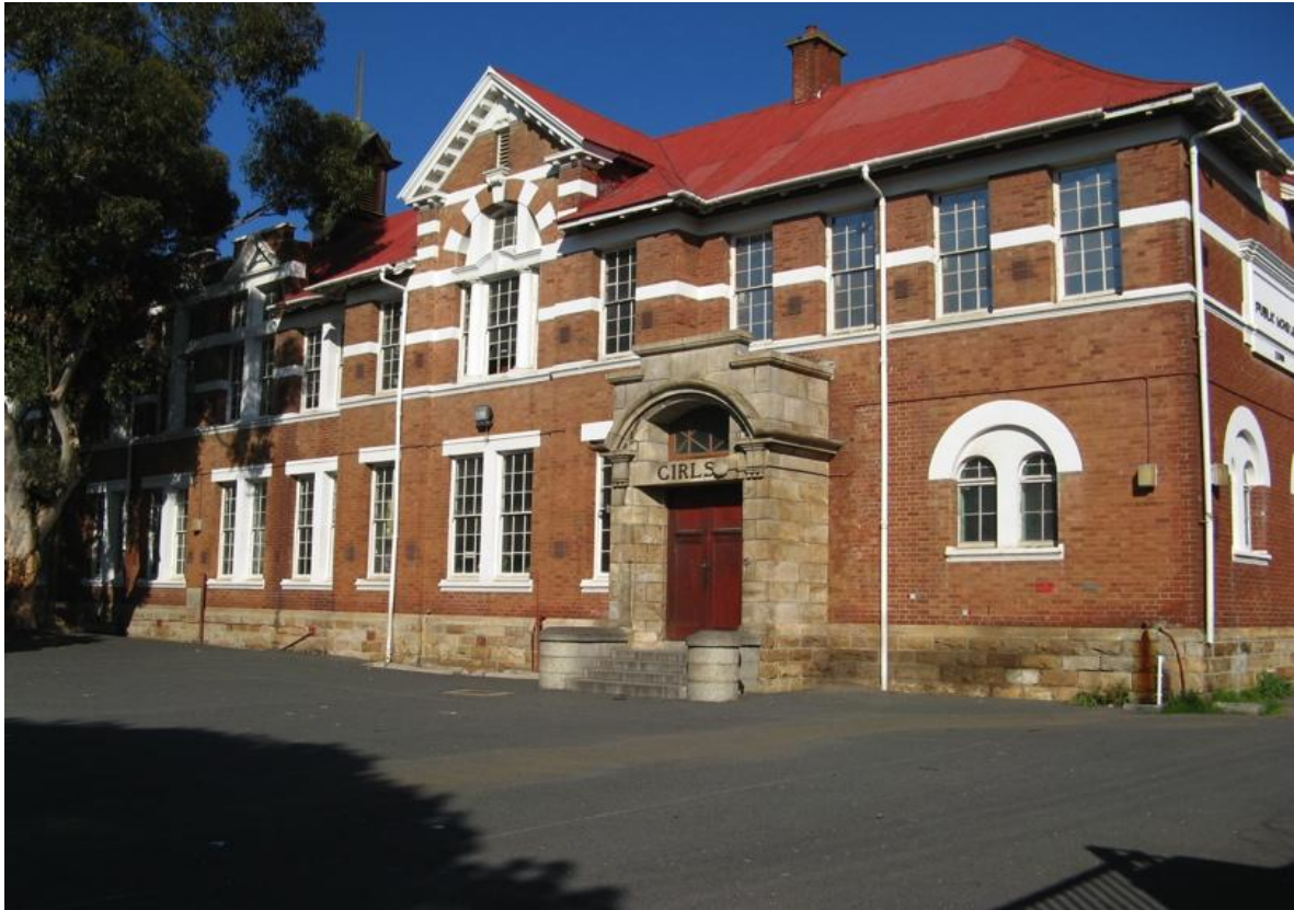
Figure 19. Prestwich Primary School (front).
