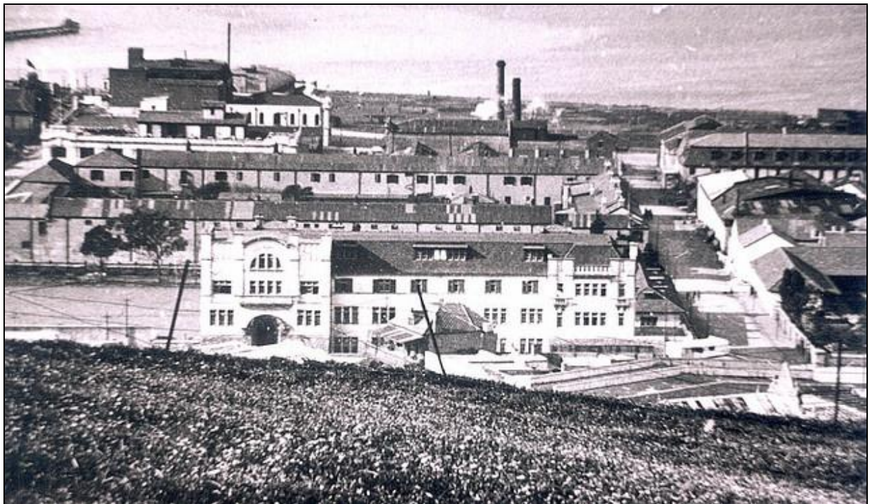
Figure 27. Picture of the Salesian Institute, Old Somerset Hospital and part of the Pavement Testing Lab. (provenance unknown).
