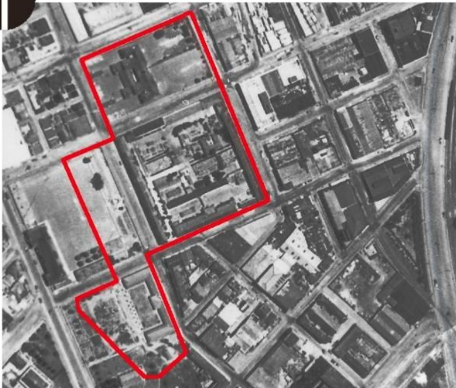
Figure 12. By 1926 the disused cemeteries were appropriated by the Municipality and the land re-used as public open space or for education/institutional purposes.
