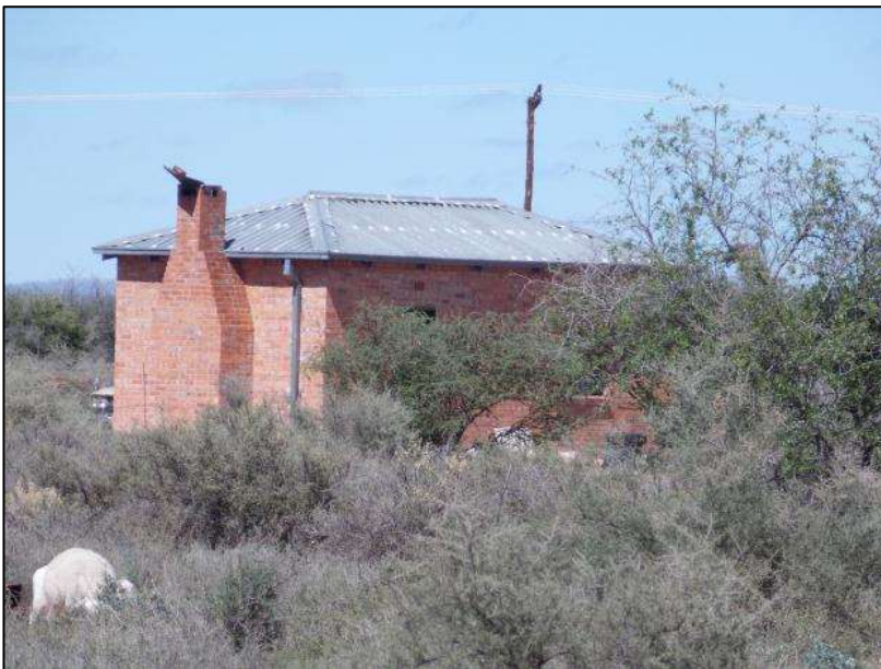
Figure 24. Labour housing on site 009
