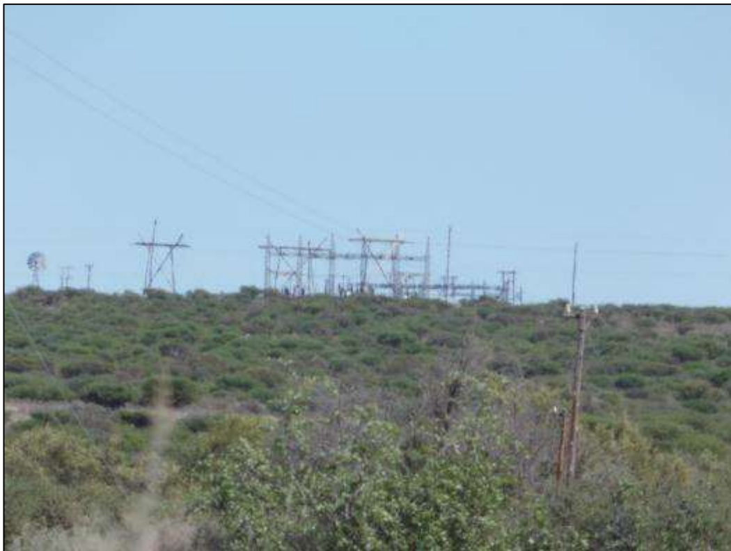
Figure 3. General Landscape and local sub-station
