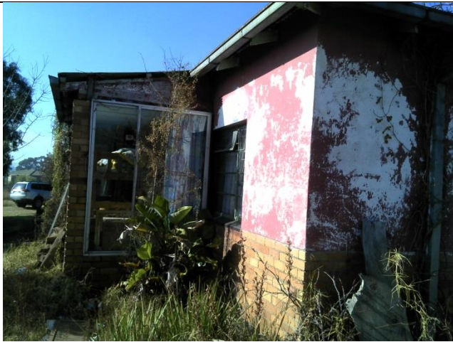
Figure 8. North western view of main dwelling.
