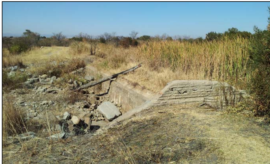
Figure 2: A section of the main dam wall
