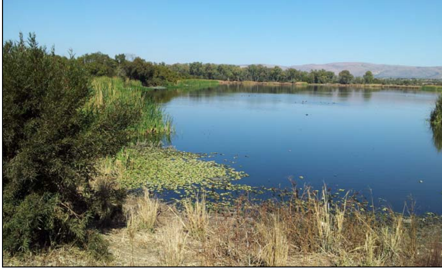
Figure 3: The extent of the dam with trees growing on the eastern dam wall
