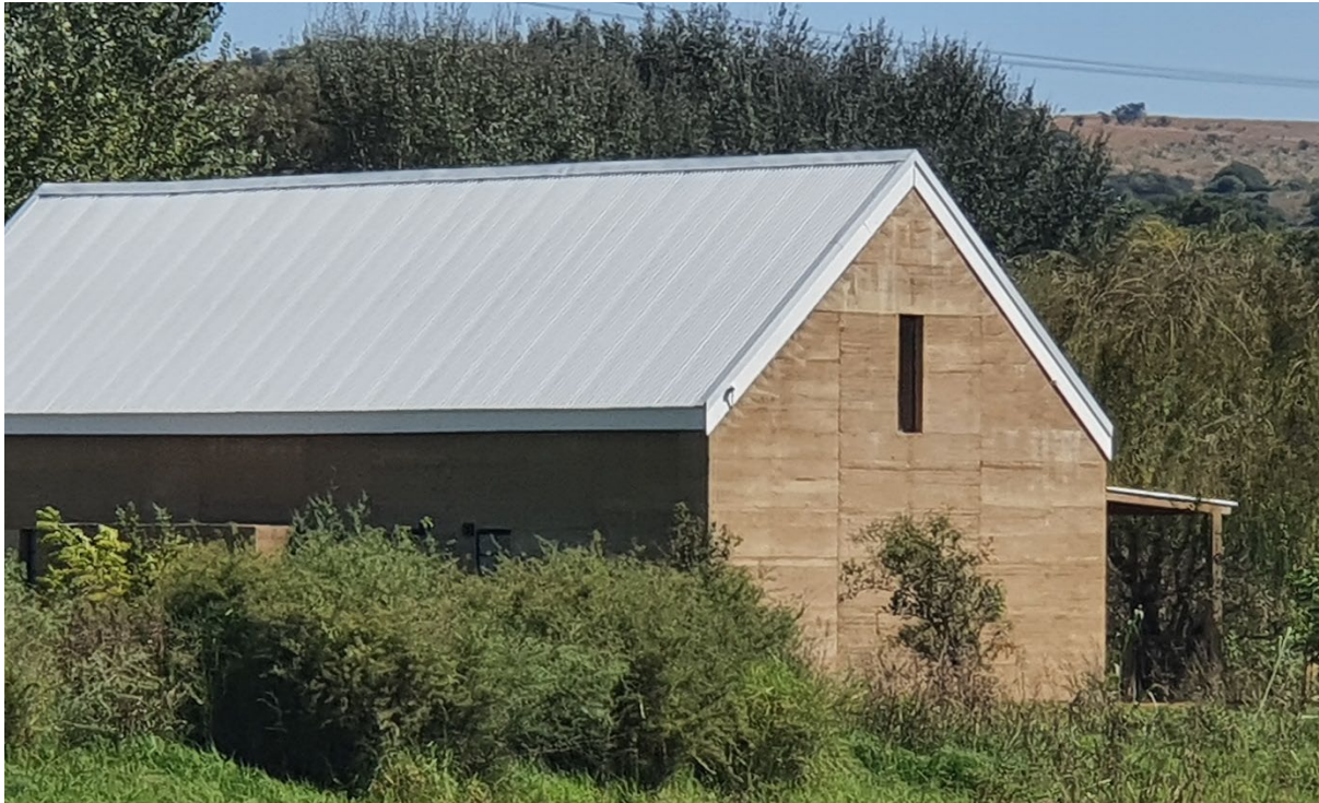
Figure 5: Proposed rammed earth building technique
