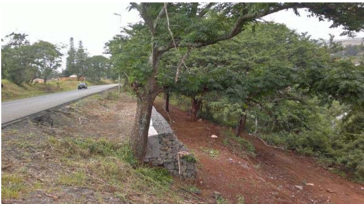
Figure 9: Road support close to pipeline route
