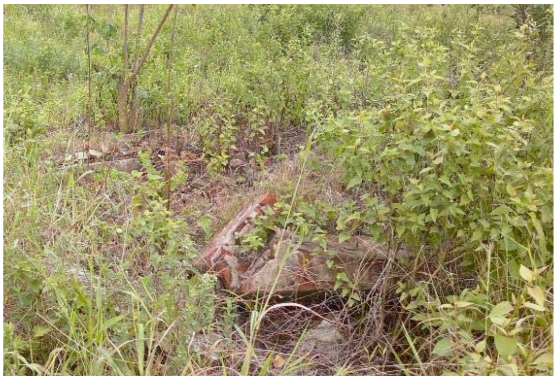
Figure 7: Remains of structure
