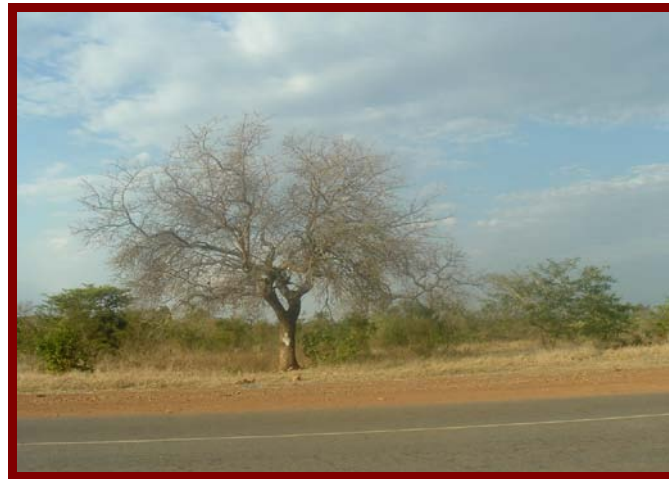
Plate 1: View of Maphophe/ Makuleke tarred road along the affected project area.
