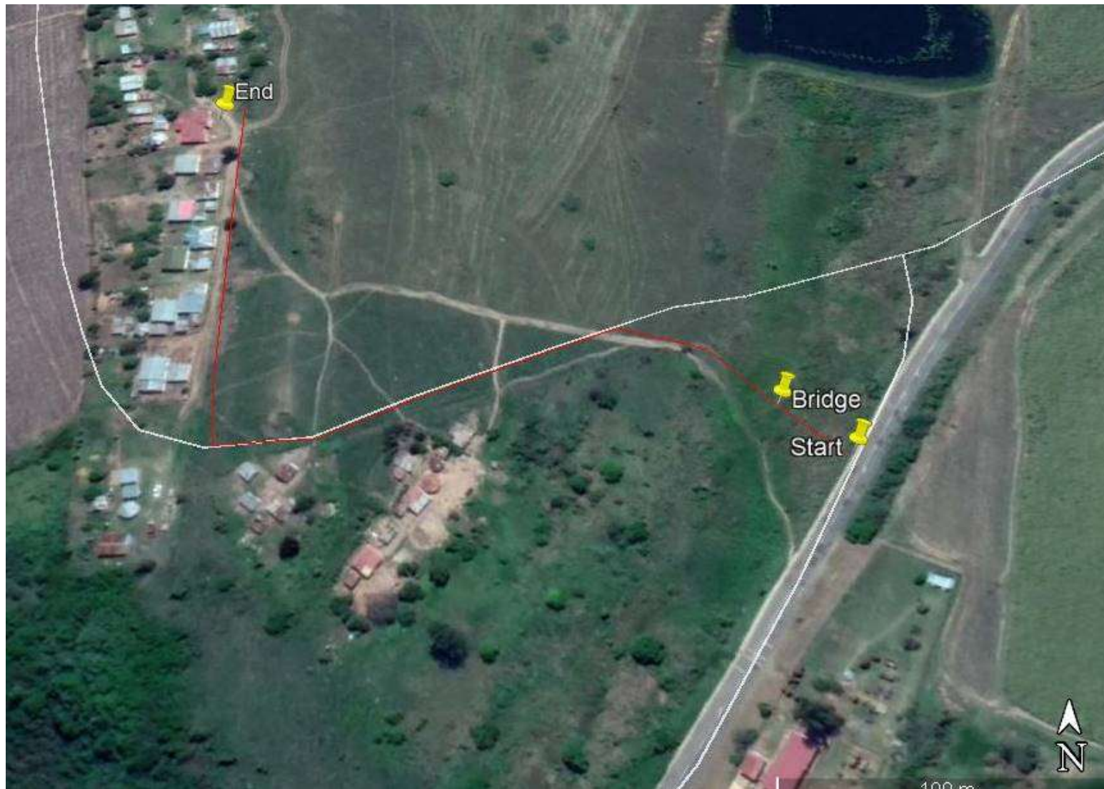
Figure 2: Closer view of road indicated in red
