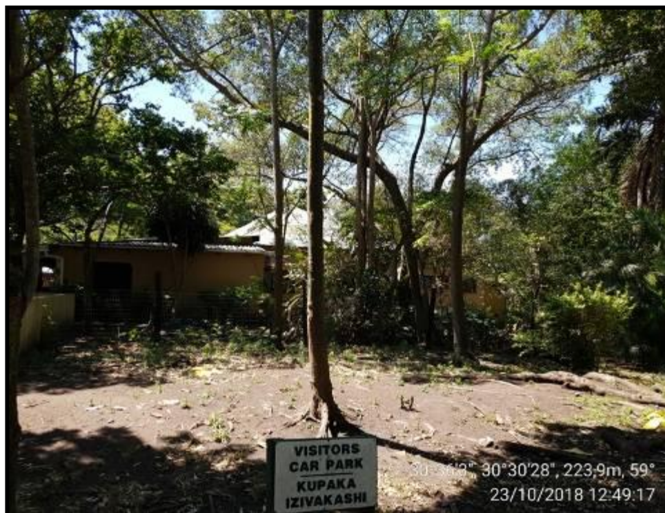
FIG. 13: THE NEUK BUILDING
