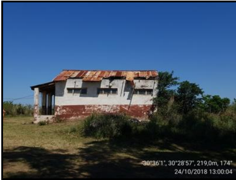
FIG. 19: GENERAL VIEWS OF THE VUKUZHAKOLE GENERAL STORE
