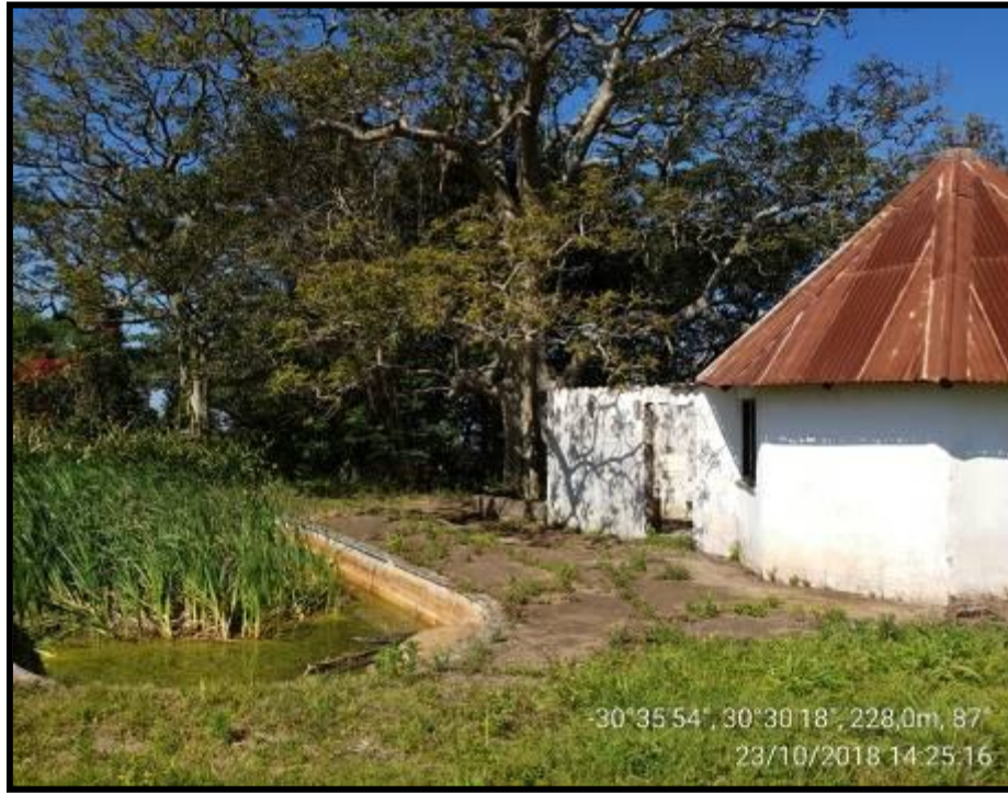
FIG. 15: RECENT BUILDINGS AT MUCKLEBRAES, THE CORNER
