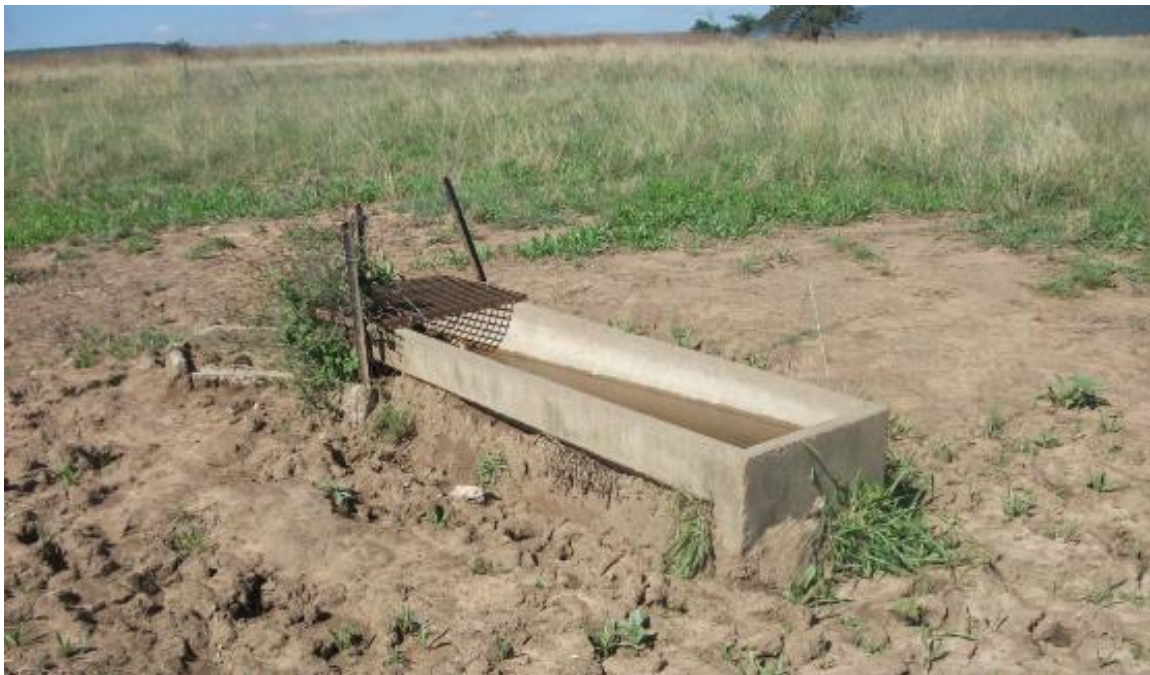
Figure 14: Cement water trough
