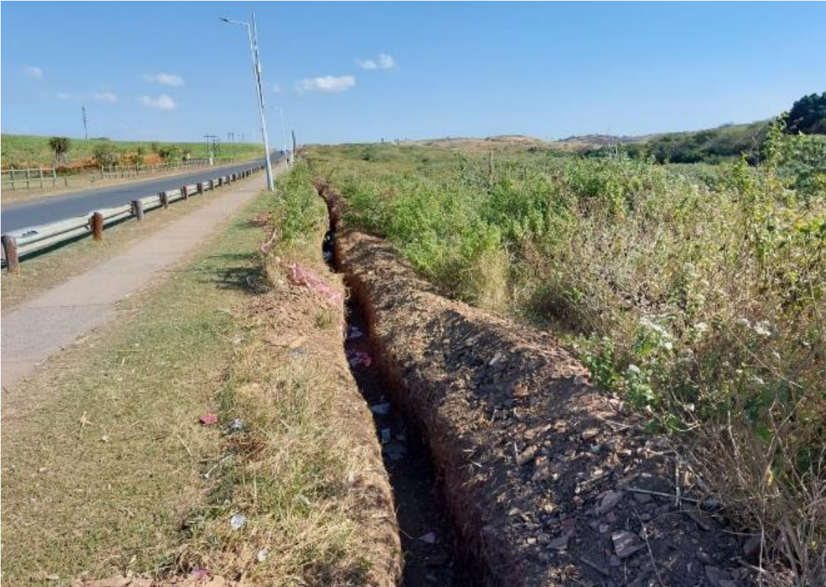
Figure 7: View of project area alongside R102 with existing trench
