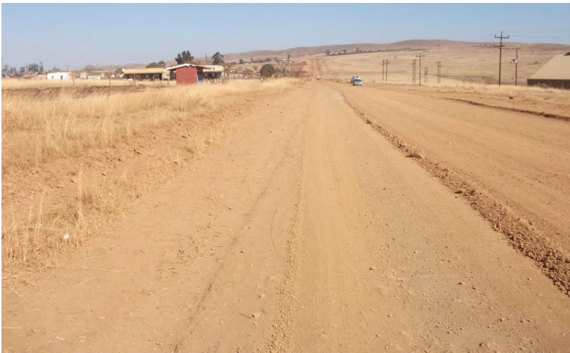
Figure 8: D1867 looking southwards
