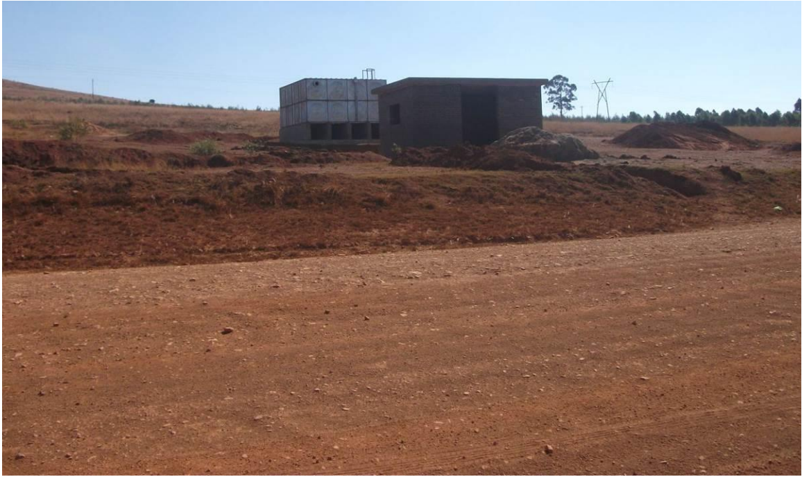
Figure 11: Reservoir and associated building
