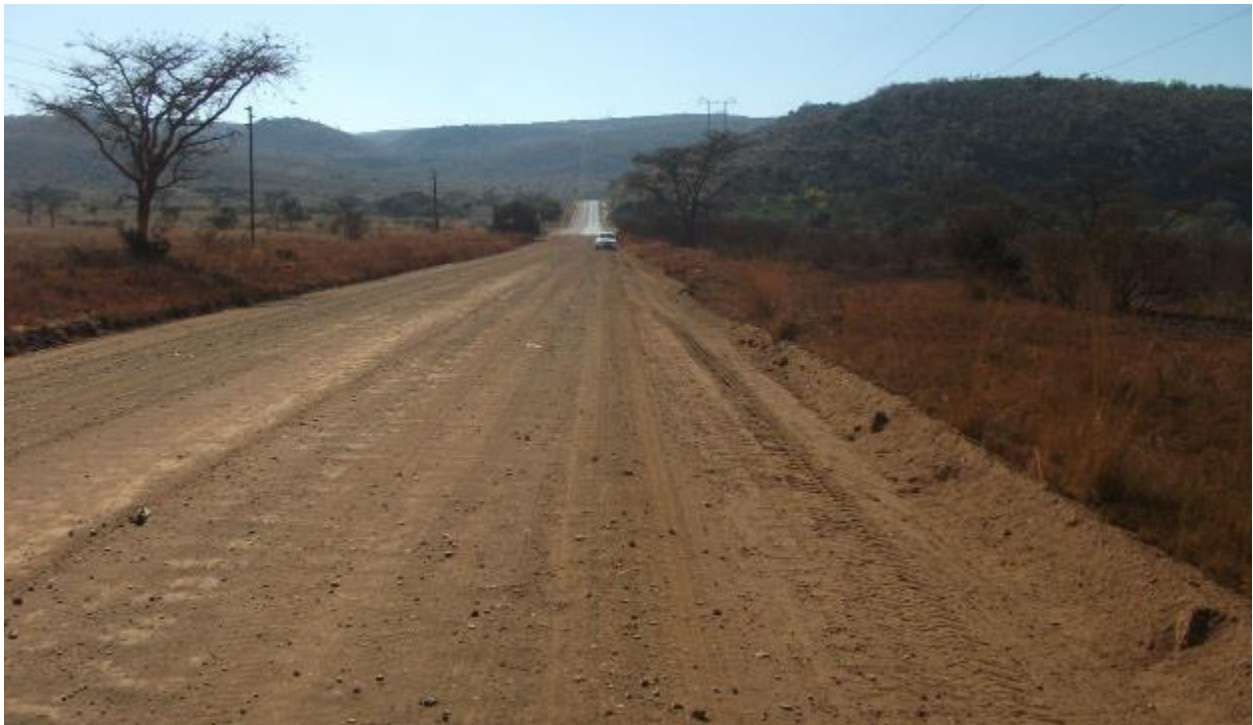
Figure 2: View towards end point of road upgrade
