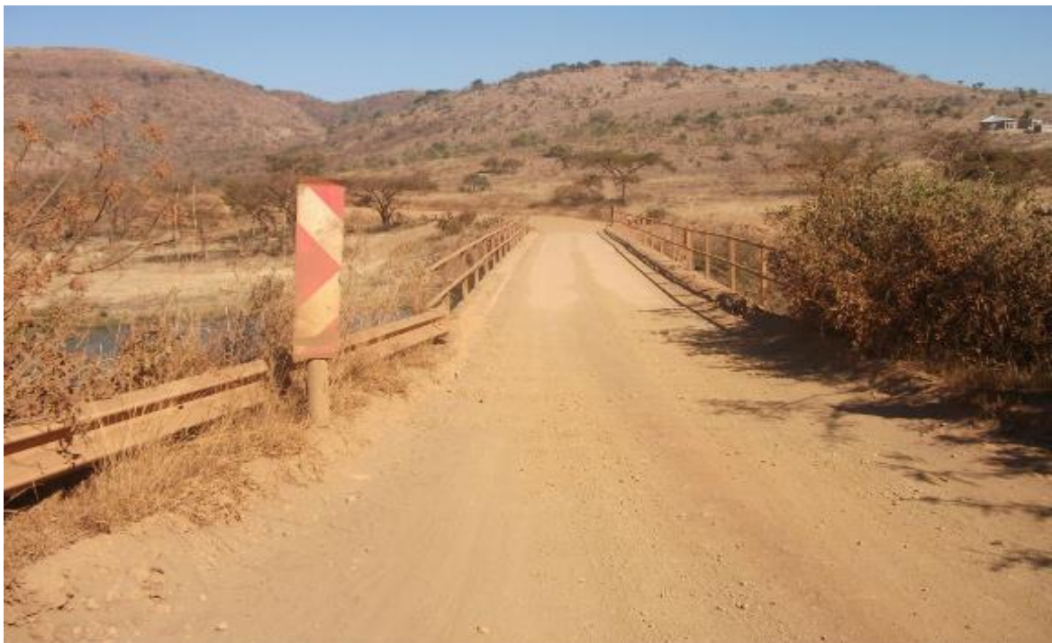
Figure 6: Existing bridge crossing Mozana River
