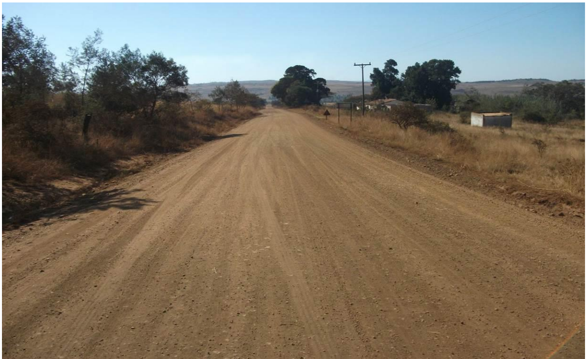
Figure 17: View of D1867 looking northwards from starting point of upgrade
