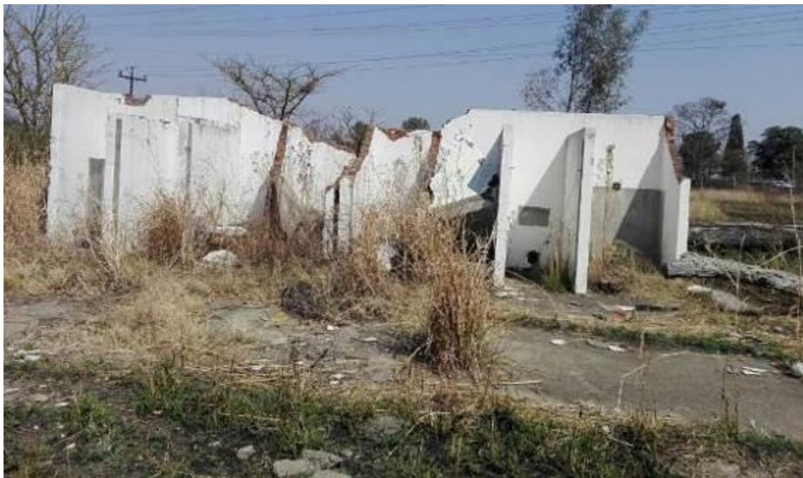
Figure 10: Dismantled ablution block
