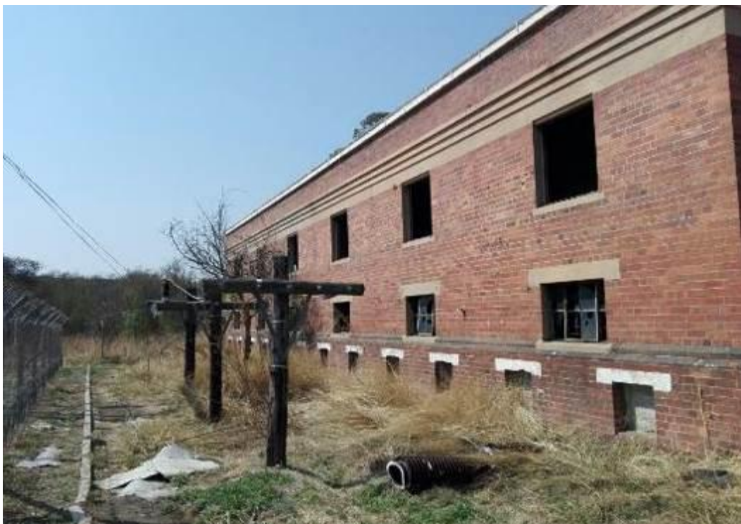
Figure 6: Power station building
