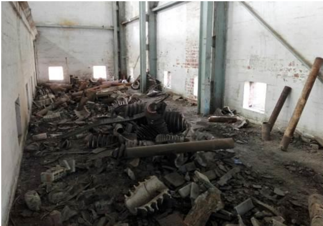
Figure 7: Interior of power station building
