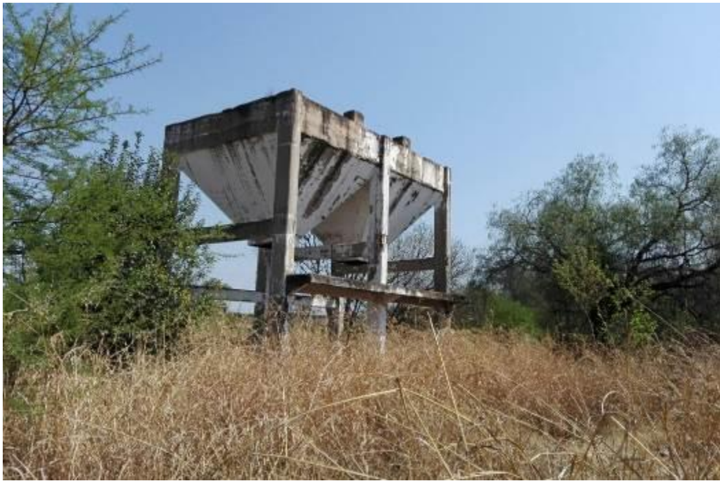
Figure 5: Intact coal hoppers
