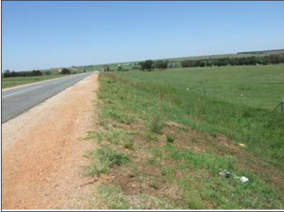
Figure 1: Road reserve of the R545 to be expanded (Photo courtesy of Martin Ferreira)
