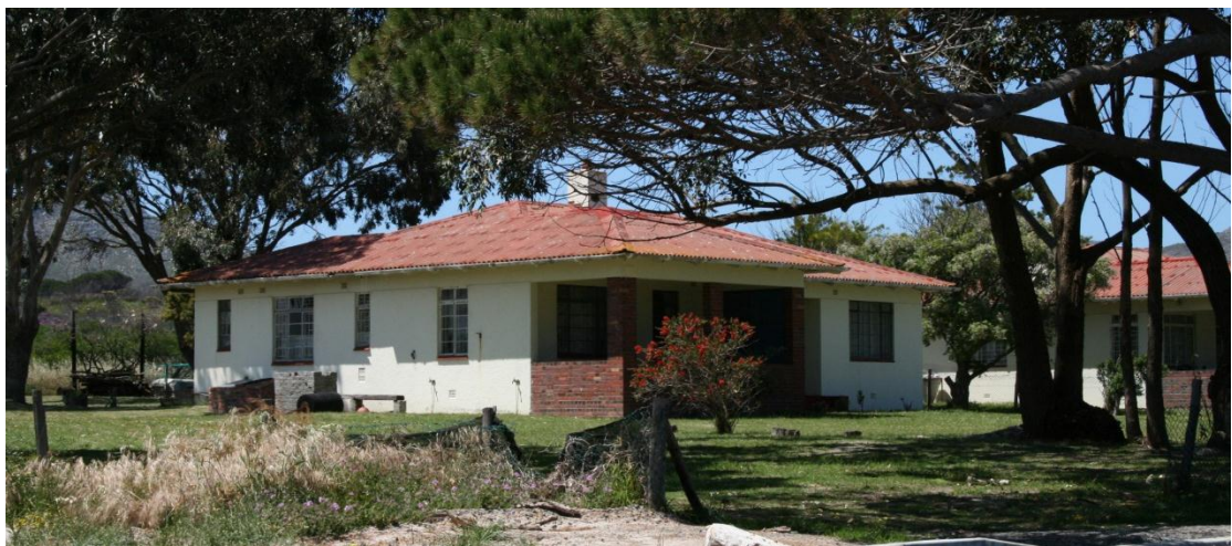
PHOTO 13: One of the houses on the Naval Radar Station site
