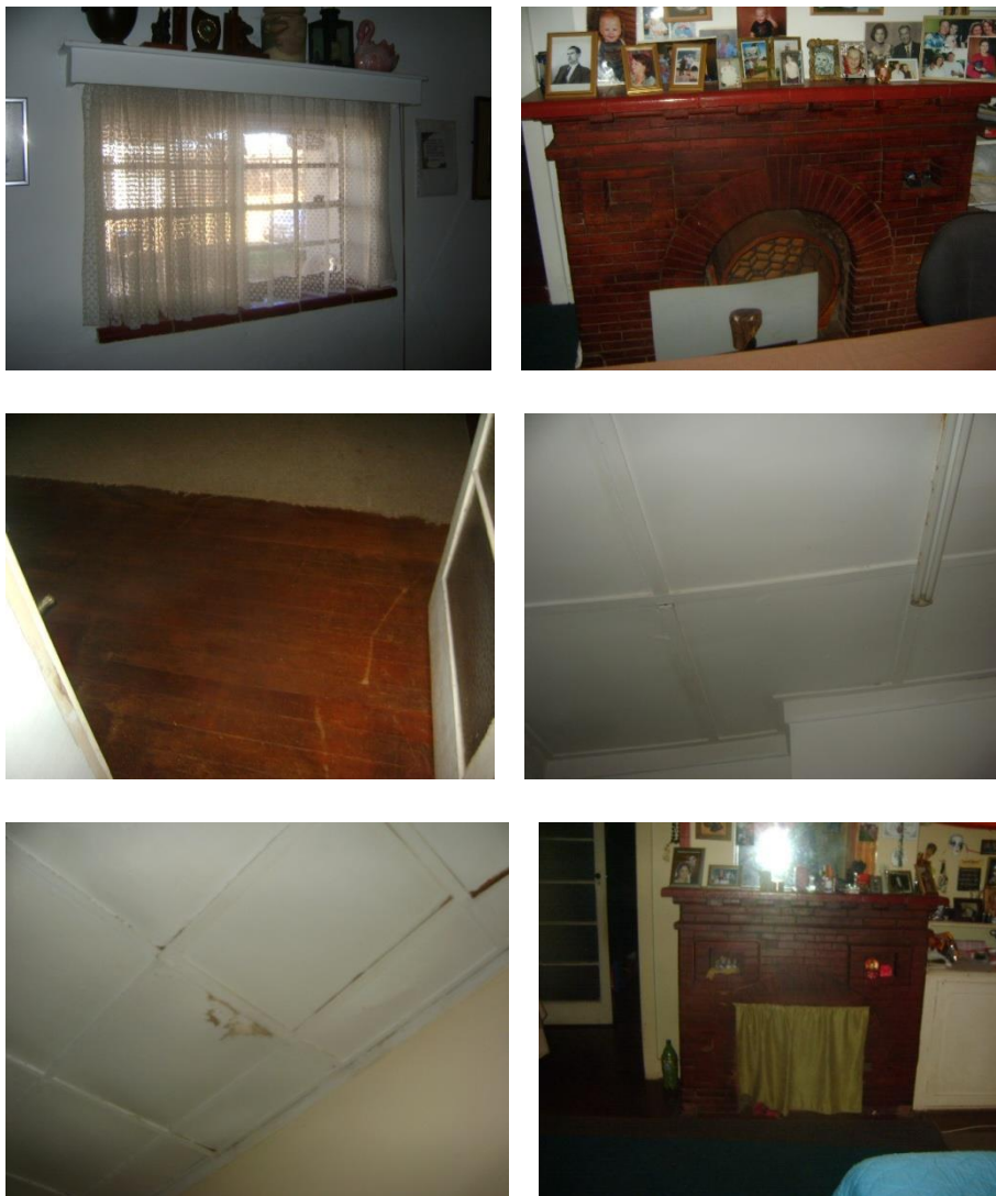
Figure 29. Images of details of windows, windowsills, fireplaces, ceiling and flooring in the old section of the building under investigation. The two red brick fireplaces are typical of the ones provided by Kirkness of Pretoria in the 1930's (Photographs S.M. Miller 2016.)
