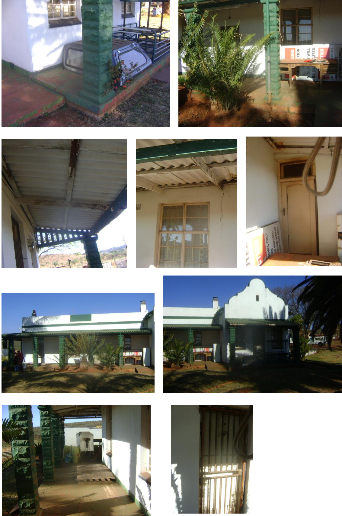
Figure 25. General views of the exterior, elevations and details of the building under investigation. (Photographs S.M. Miller 2016.)
