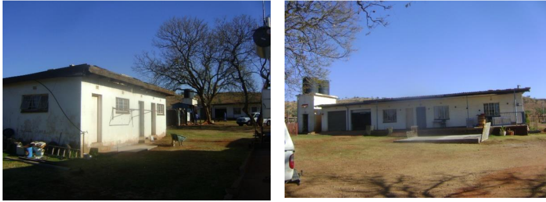
Figure 23. Above are the two unprotected modern buildings surrounding the building under investigation. (Photographs S.M. Miller 2016.)
