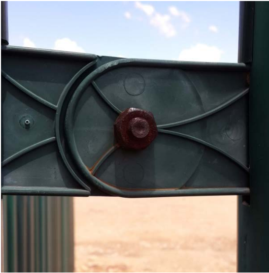
Fig 3 : weak connector between fence
