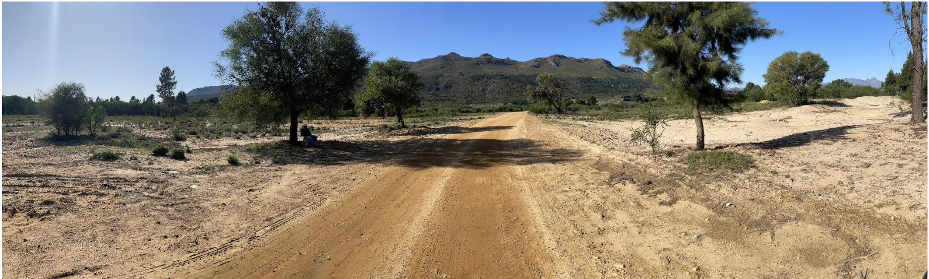
View looking east along the internal road of the site from the western boundary
