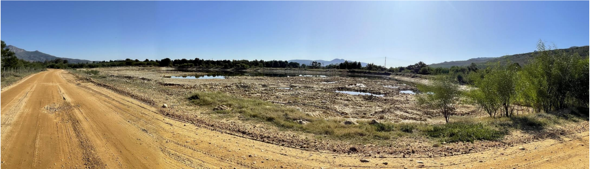
Stitched photograph of the excavated area in the middle of the site
