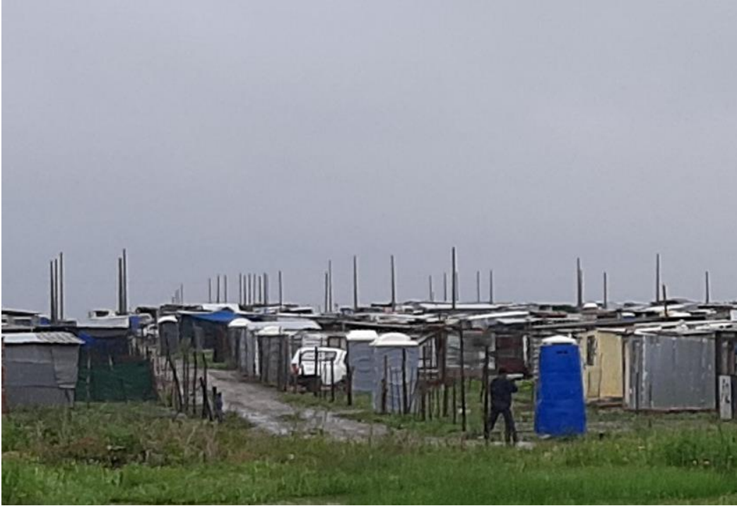
Figure 3: Informal houses at Putfontein
