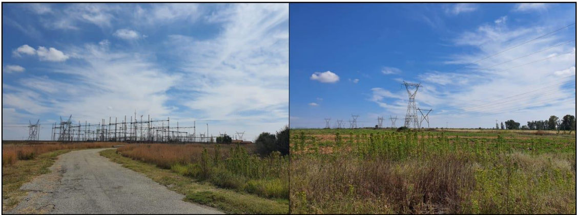
Figure 5-7: View of the western offset of the project at the Eskom substation (left) and the project corridor through cultivated land (right).
