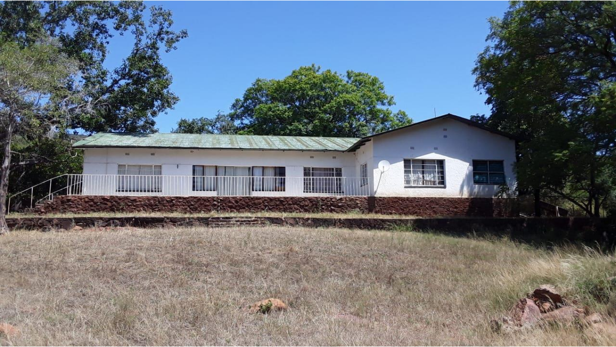
Figure 18: View of River House.
