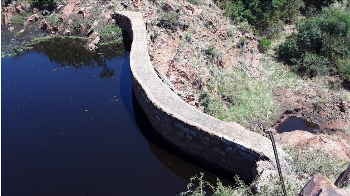
Figure 20: Dam located close to the proposed Spa complex.
