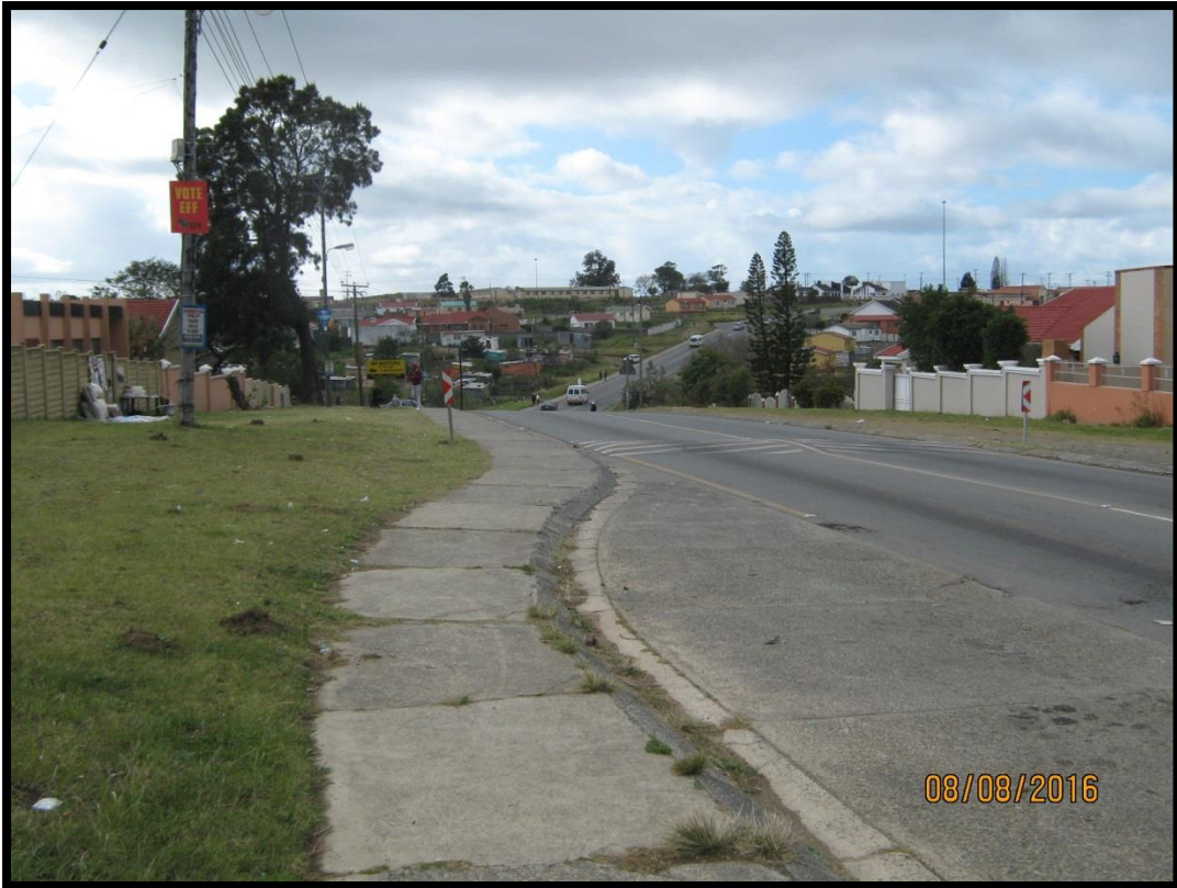
Figure 10: Road with shoulder covered in grass. View to the west. Position of culvert 3.
