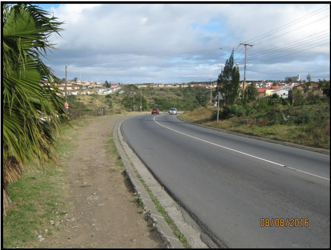
Figure 13: Road and shoulder to the east. View towards culvert 1.
