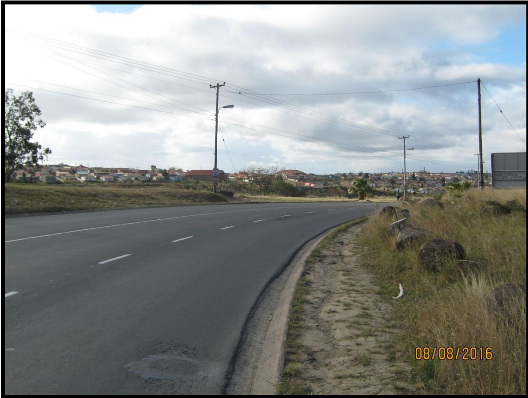
Figure 14: East view on pavement at 4.2 km.
