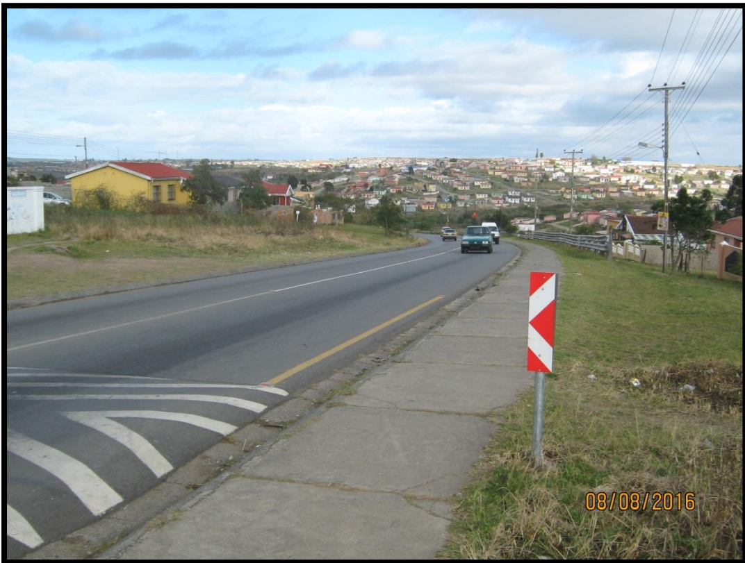
Figure 11: Road and shoulder to the east. View towards culvert 2.
