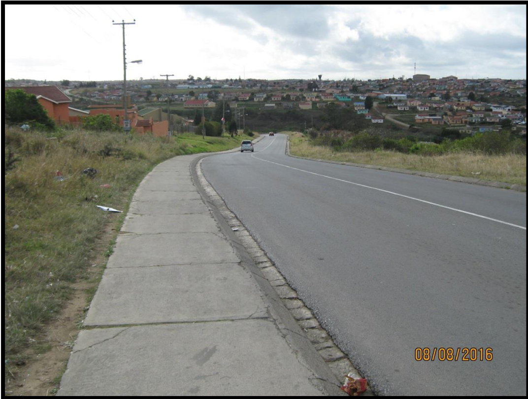
Figure 12: Road and shoulder to the east, sandstone is visible.
