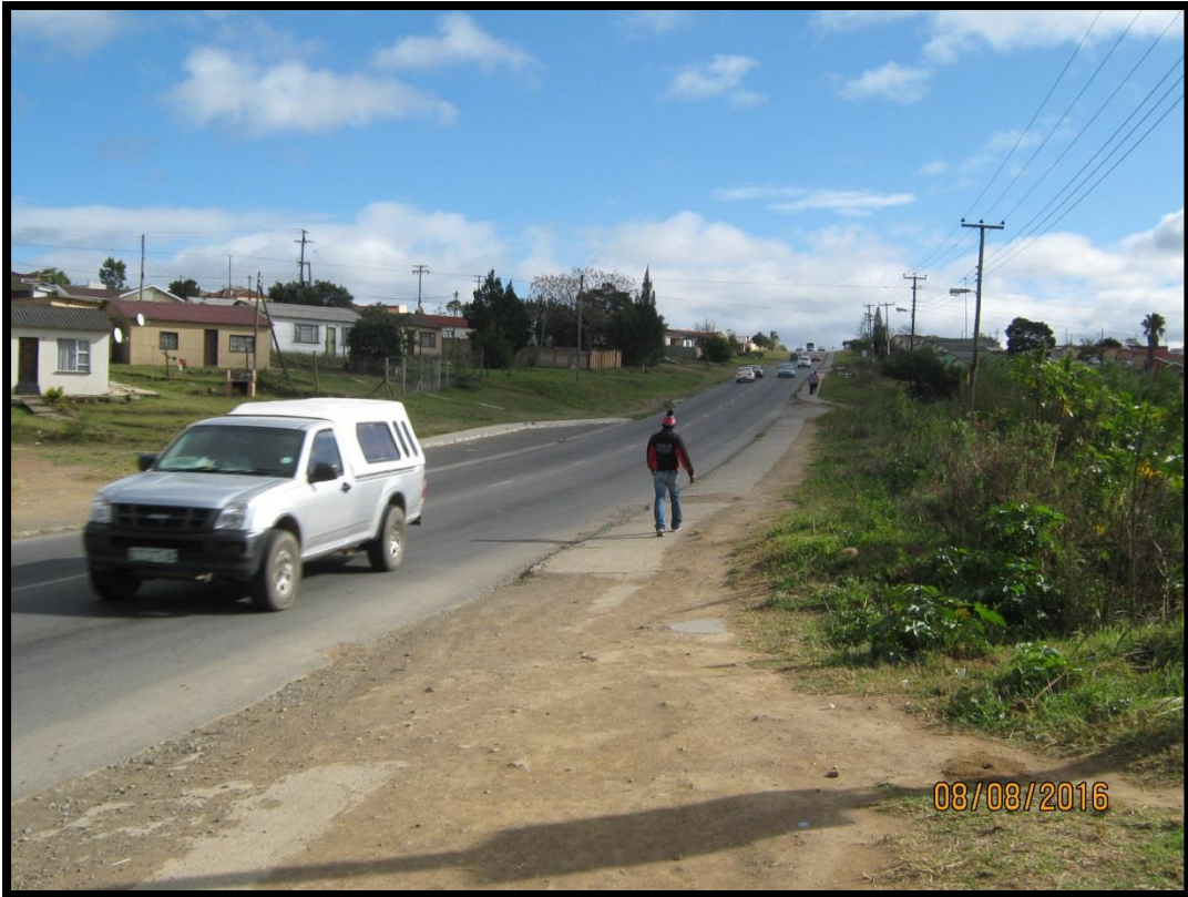
Figure 8: Example of a mudstone found near petrol filling station and beginning of road upgrade (S 28°21'645", E 28°22'985"). This type of outcrop will need mitigation as it is right on the shoulder of the road.
