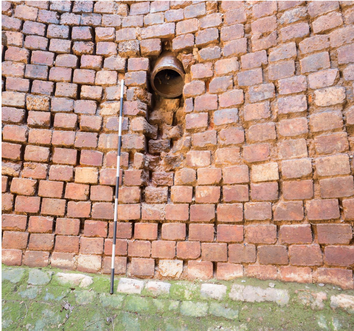
Figure 49. Modification of the kiln by introduction of a coal chute. There is no vitrification of the brickwork or pipe and it is unlikely that the intervention ever worked.
