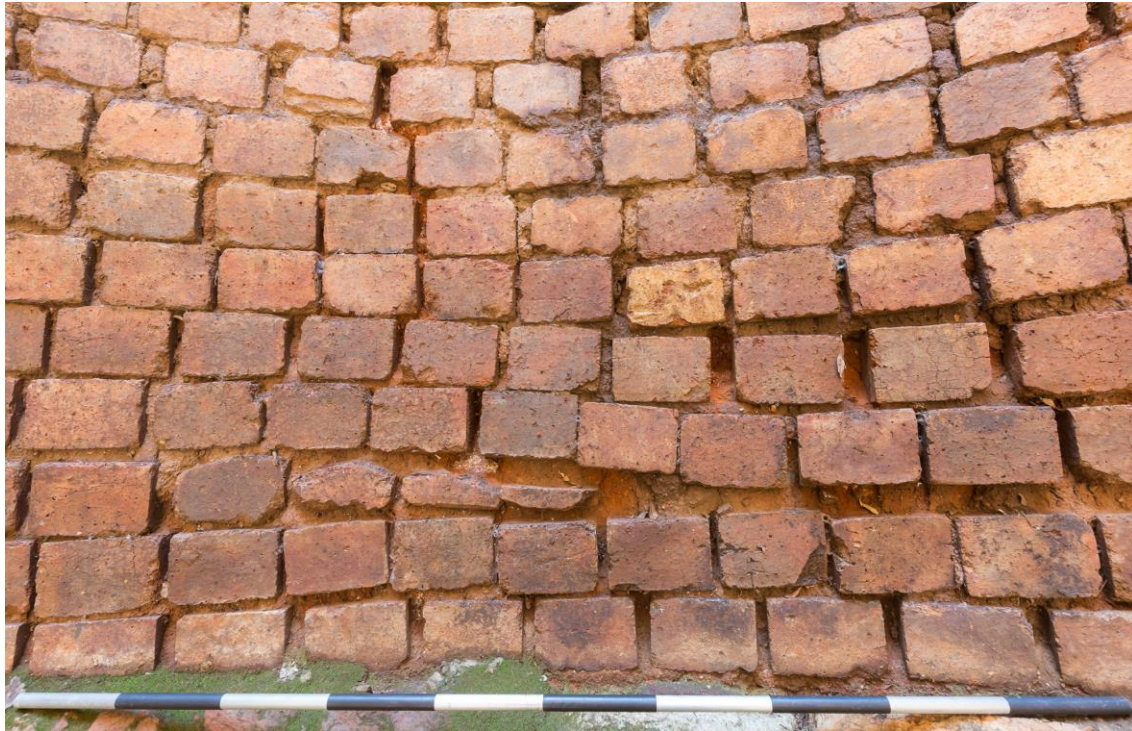
Figure 42. Detail of the brick coursing of the vertical lining of the kiln.
