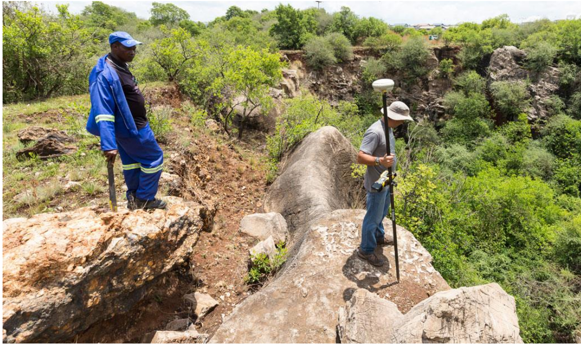
Figure 22. Area where overburden has been excavated behind a large dolomite boulder on the edge of the quarry.
