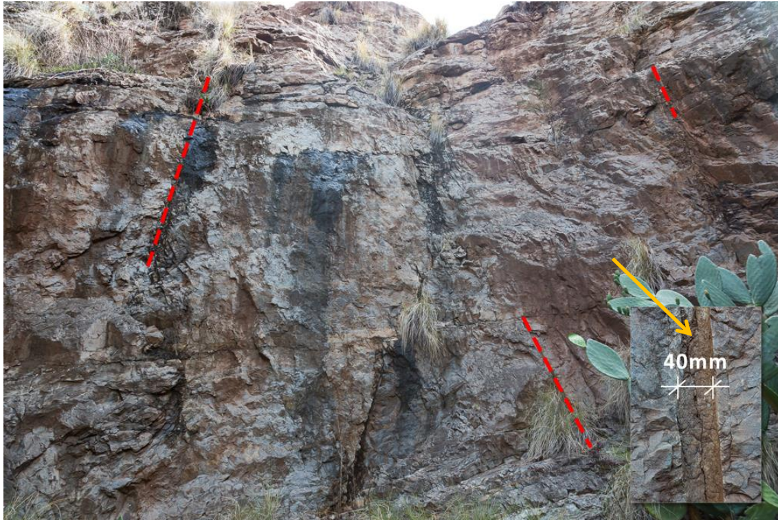
Figure 23. Drill marks on a vertical wall of a quarry. Also see insert showing scar width.
