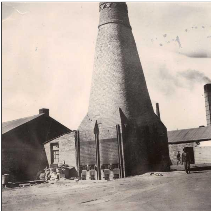
Figure 8. A brick downdraft kiln at Olifantfontein used in the production of ceramics by the Ceramic Studio ( http://www.artefacts.co.za/ ).
