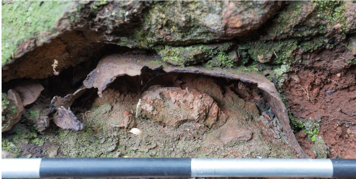
Figure 47. Remains of a steel railway sleeper used as a lintel.
