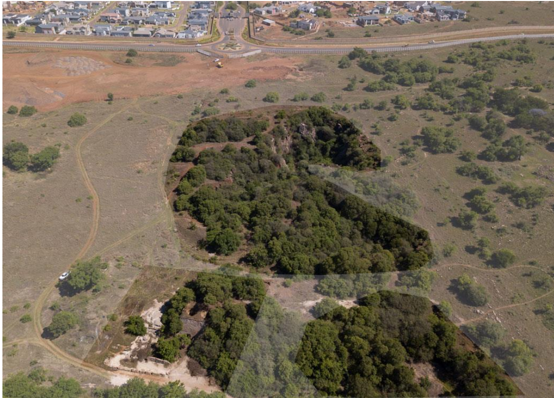
Figure 17. General view of the quarries showing the production area at the bottom left.
