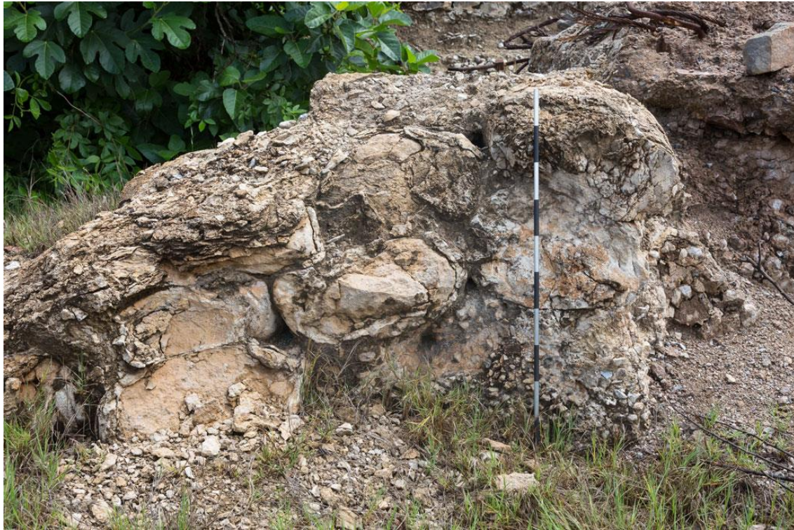
Figure 57. Ramp-like structure made of lime-filled hessian bags. Note the cables imbedded in the structure on the right.
