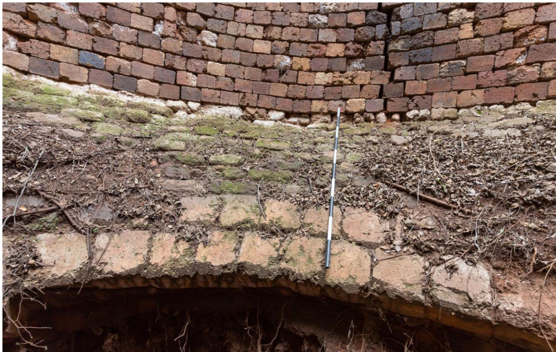
Figure 43. Detail of the firebrick used at the centre of the kiln base. The first few rows were lined with ordinary fire bricks but the fire-bricks in the last two rows have different dimensions. The bricks are 160 x 140 x 200 mm in size.
