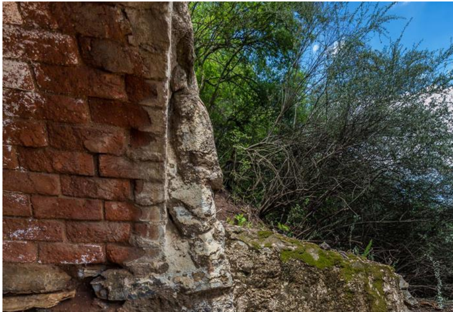
Figure 39. Detail of the exterior stone cladding and brick vault joint.
