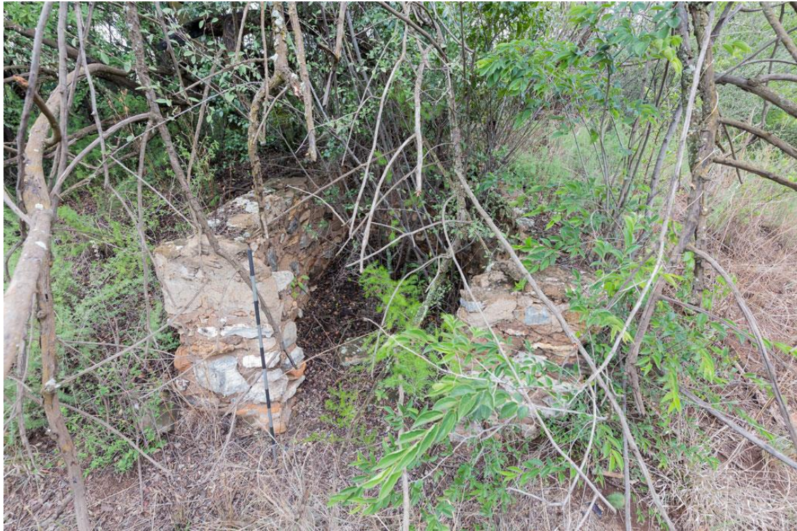
Figure 24. Remains of an explosives-holding area along the northern edge of the quarry.
