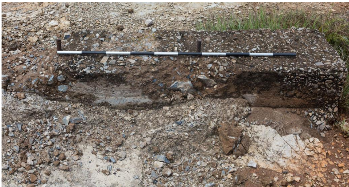
Figure 58. Mounting block for machine showing a flywheel imprint and hydrated lime residue. This was presumably a mechanical screen with an offset flywheel to vibrate the screens.
