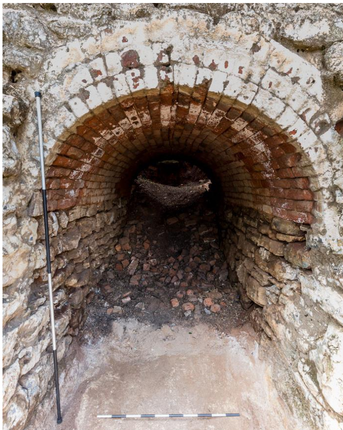
Figure 37. Detail of the kiln entrance showing the rock and brick construction. Note the lime floor and debris that have accumulated in the interior of the kiln. The scale on the ranging rod on the left is demarcated in 500 mm sections with a total length of 2000 mm.
