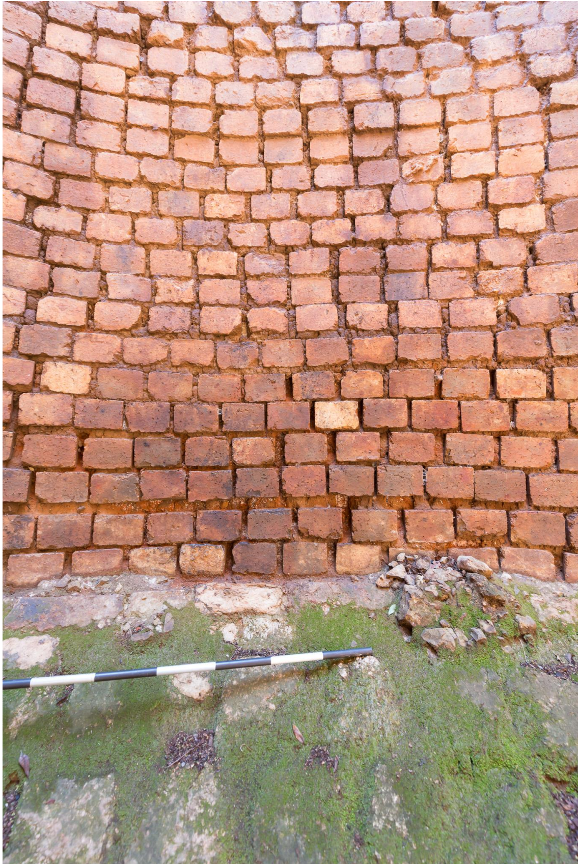
Figure 41. Detail of the joint between the vertical kiln lining and the kiln base. Note the few lumps of unburnt limestone that remain on the kiln base.
