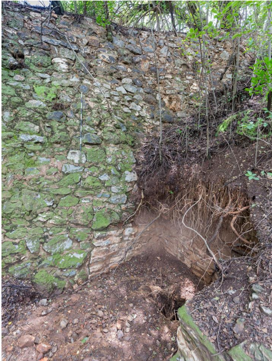
Figure 48. Retaining ramp constructed over the second draw hole.
