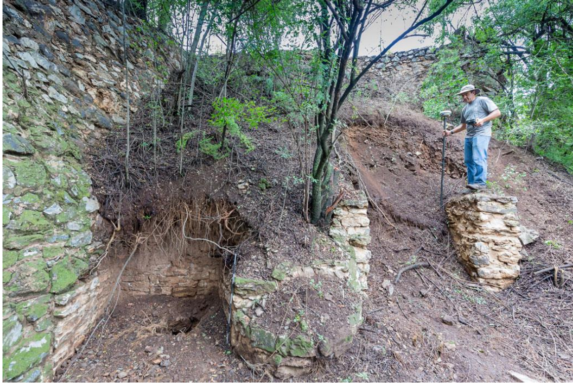
Figure 45. Additional draw holes likely constructed at a later stage.
