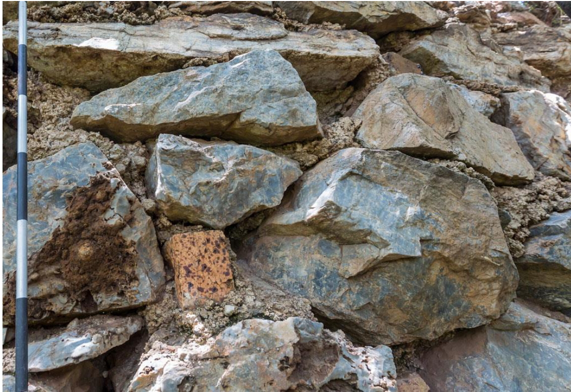
Figure 52. Another example where repairs were undertaken on the south-western corner of the kiln. Note the Cullinan brick in the wall.
